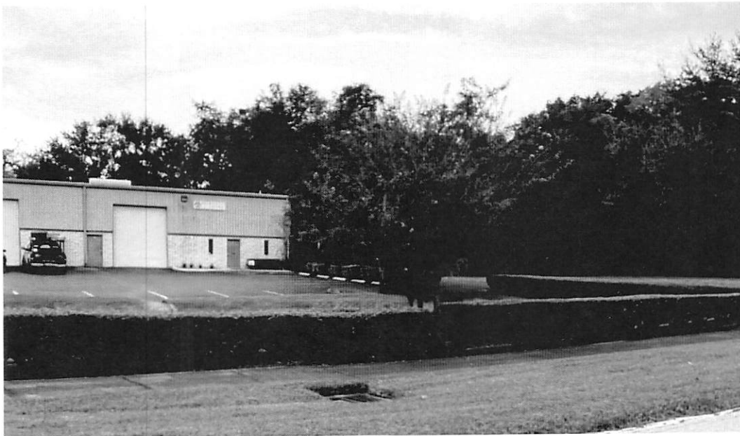
Property to the east
