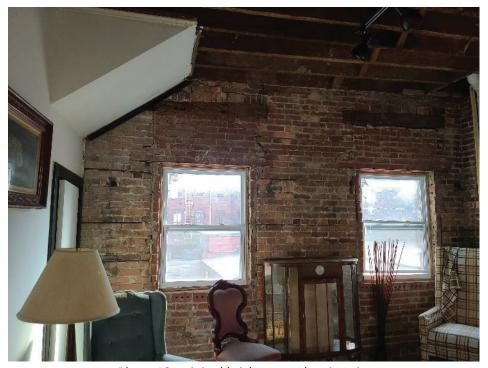
Photo 10, original brick exposed on interior
