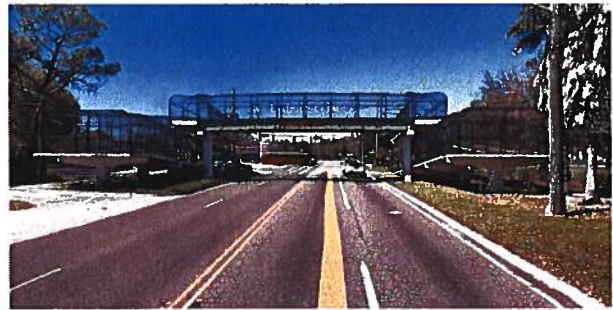
Moncrief Road Pedestrian Bridge
