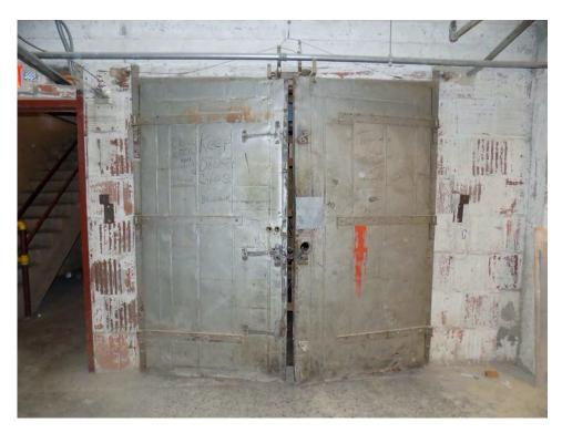
Photo 28 - Interior, basement Unit E, elevator fire shutter door, looking east.
