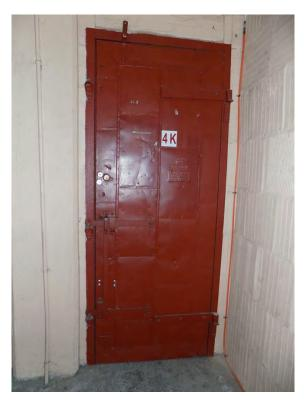
Photo 30 - Interior, fourth floor Unit K, fire shutter door from stairwell, looking east.
