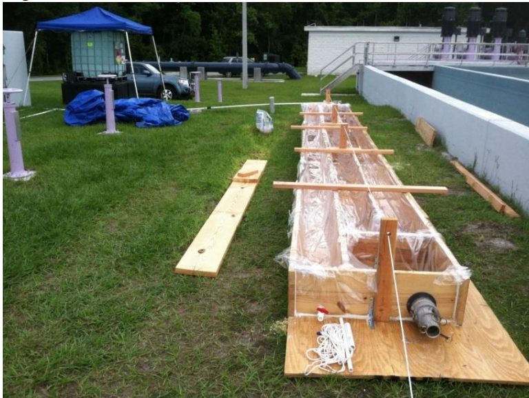
Figure 5 – CCUA Model Chlorine Contact Chamber Under Construction
