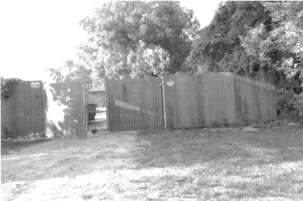
View of existing fence on Boulder Street
