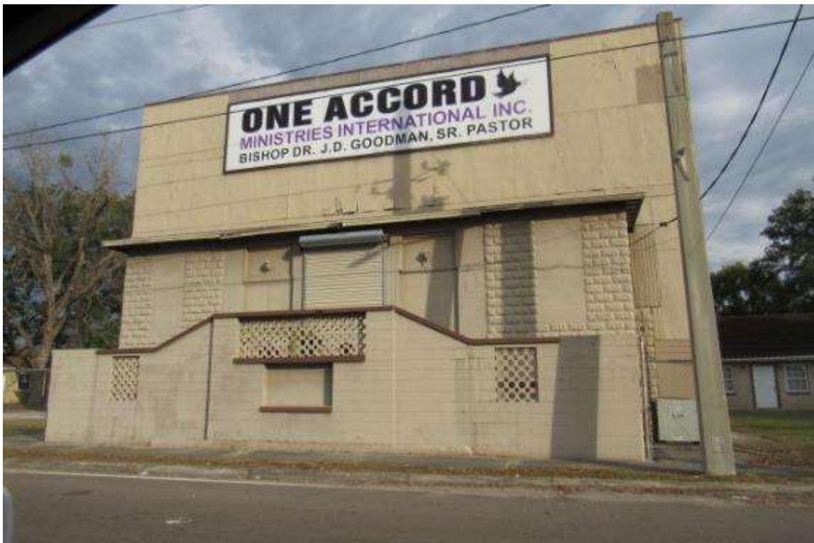
Existing church building
