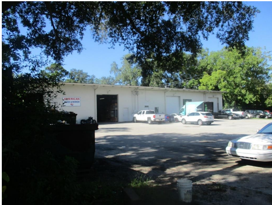
View of the neighboring glass and mirror business to the west of the subject site along Clydo Road.
