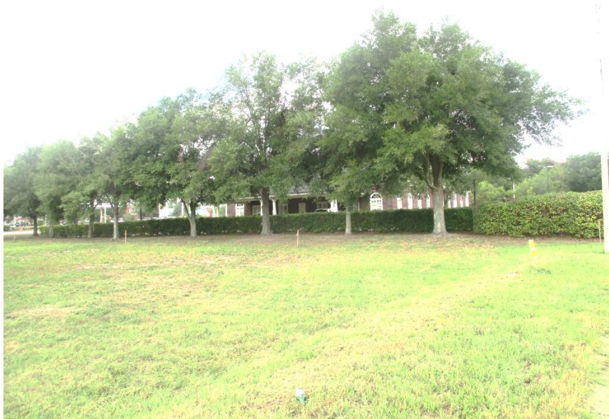
View of the office structure to the west.
