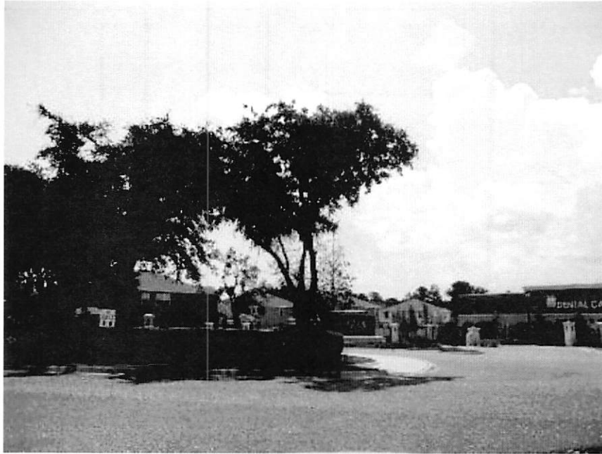
View looking south toward the single family subdivision from the south western portion of the subject site.
