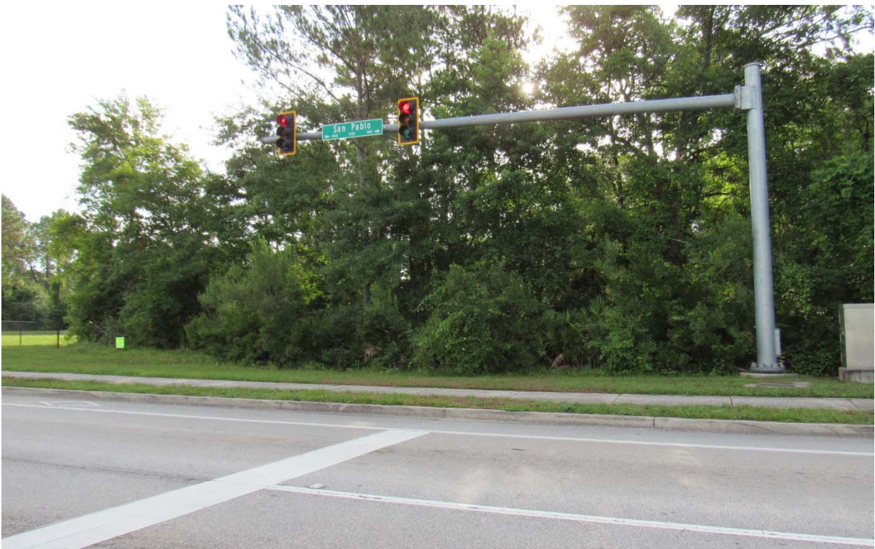
The subject site facing east from San Pablo Pkwy.
