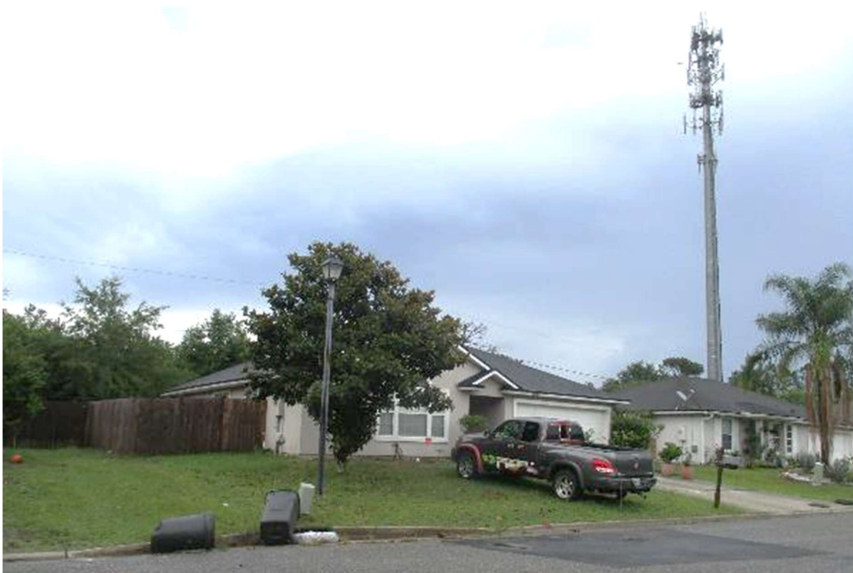
Existing cell tower on subject property.
