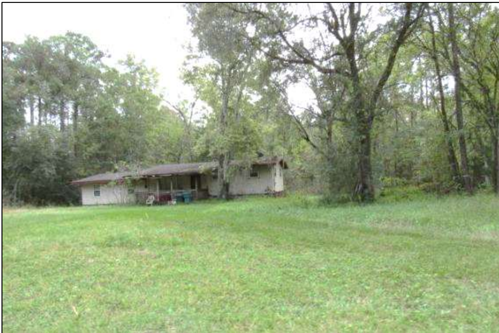
Abandoned house on subject property
