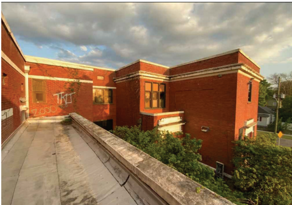
Exterior of building facing southeast
