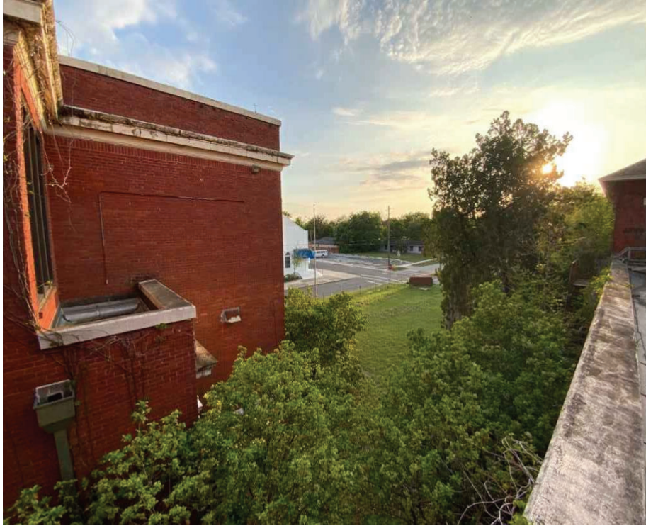
Exterior of building facing southwest
