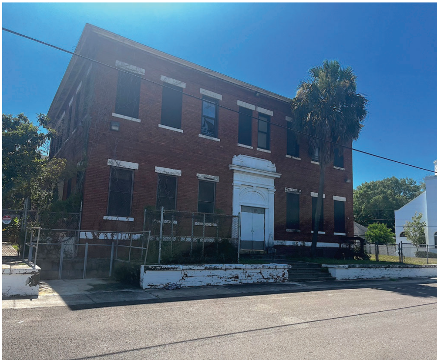
Front of Building – West Entrance
