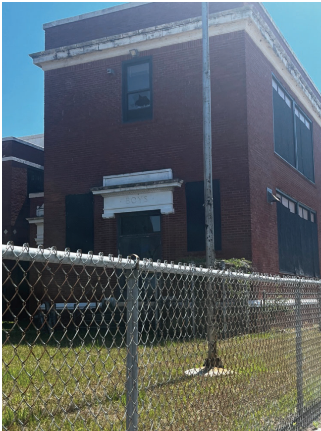
Southwest Corner Closeup
