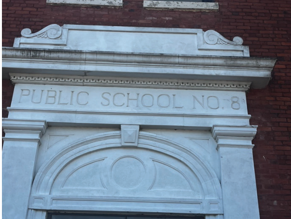
West Entrance Close up
