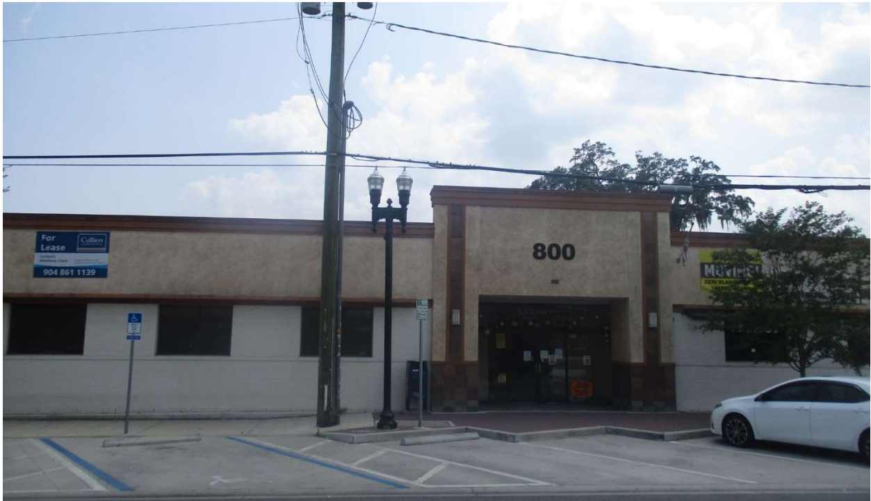
Source: Planning & Development Department, 07/19/2023
