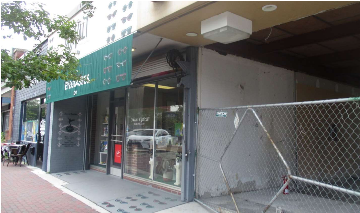
Source: Planning & Development Department, 07/19/2023
