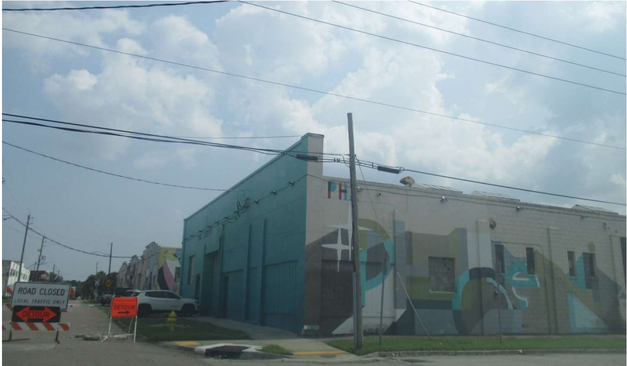
Source: Planning & Development Department, 07/19/2023
