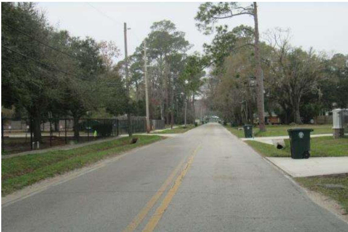
View of Livingston Road and drainage swales
