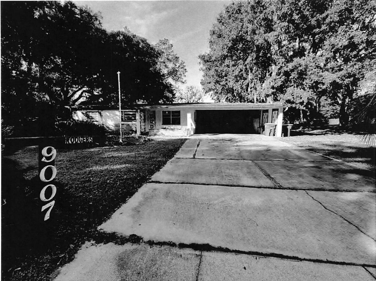
Source: Planning & Development Department 11/8/2022 View of property 9007 Noroad
