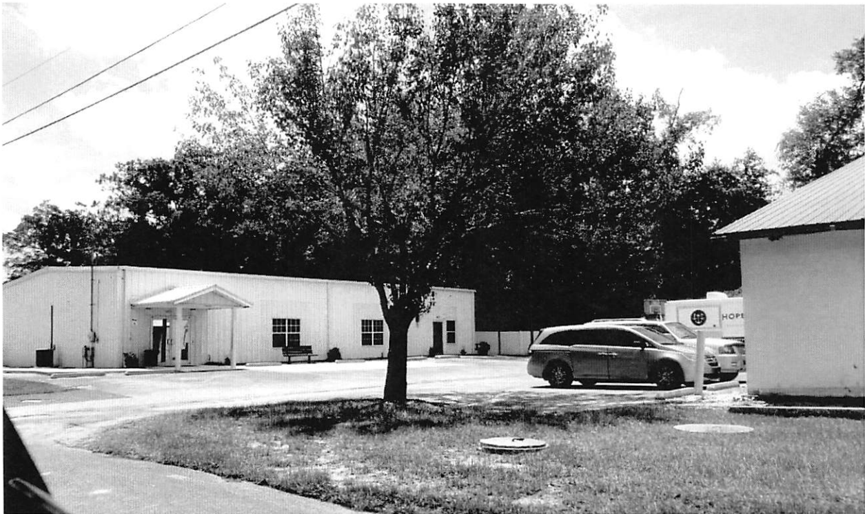
Source: Planning & Development Department, 07/13/2022 View of the subject property.
