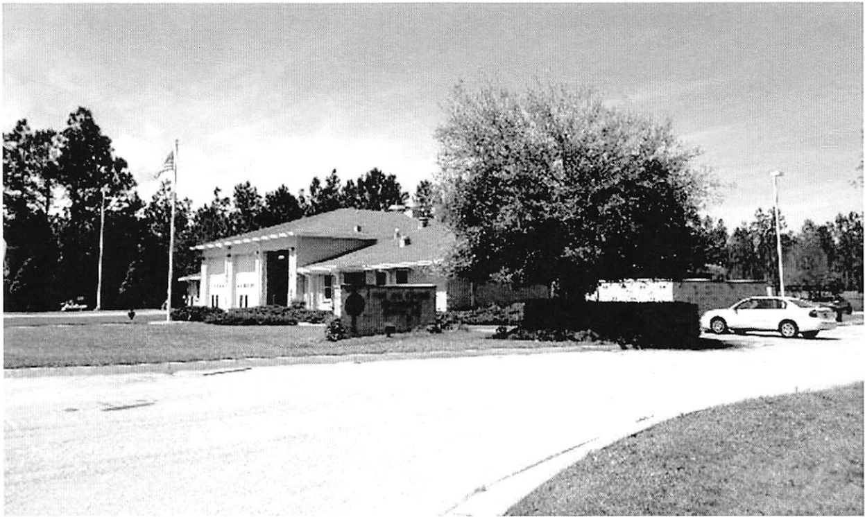
COJ fire station adjacent to proposed development.
