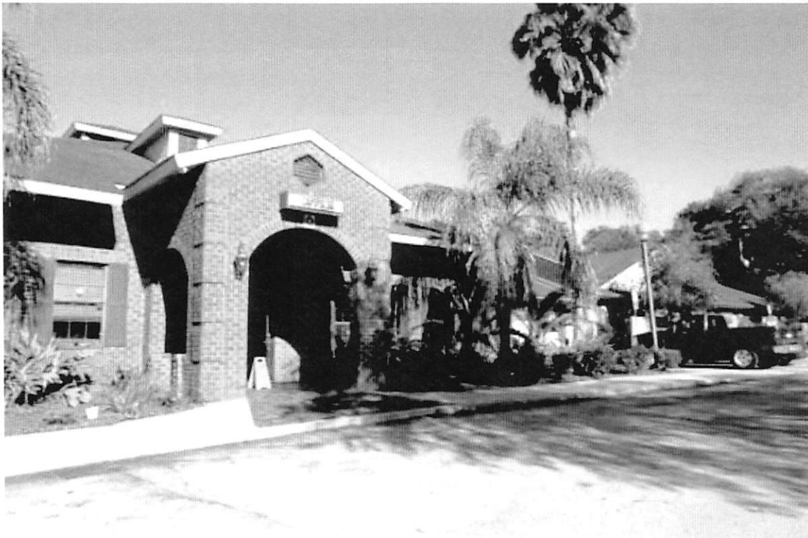
View of motel building
