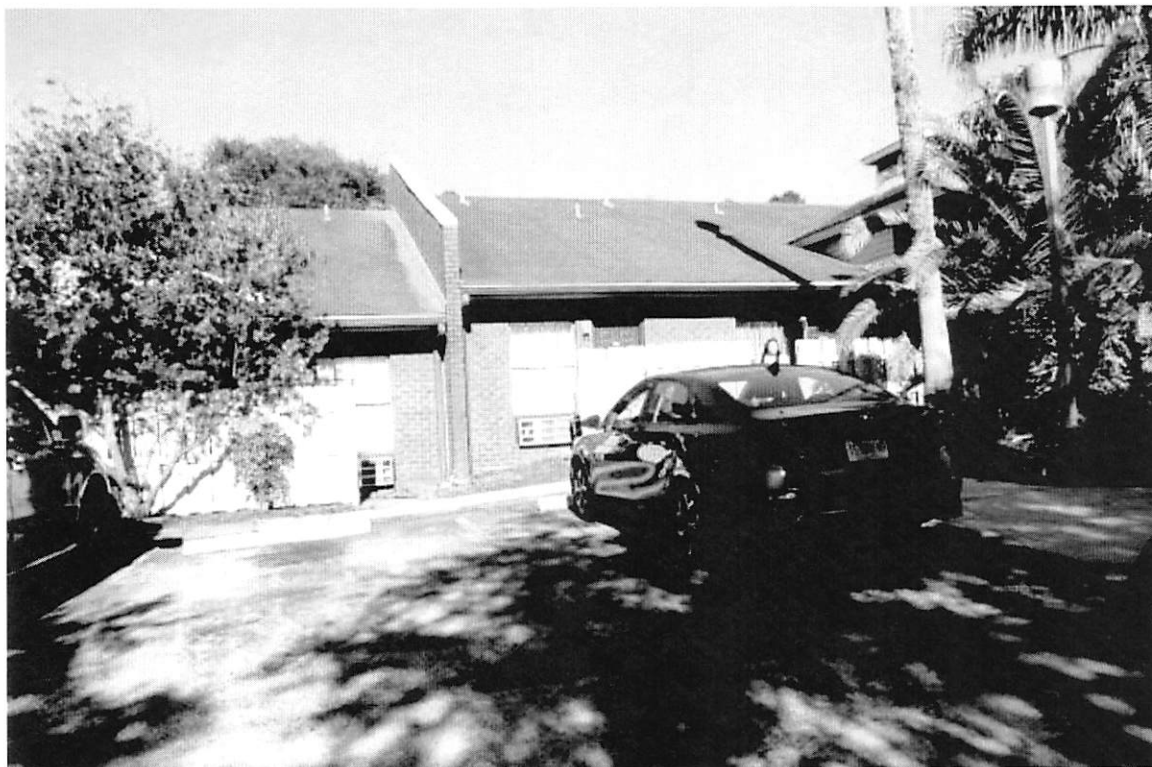
View of motel building
