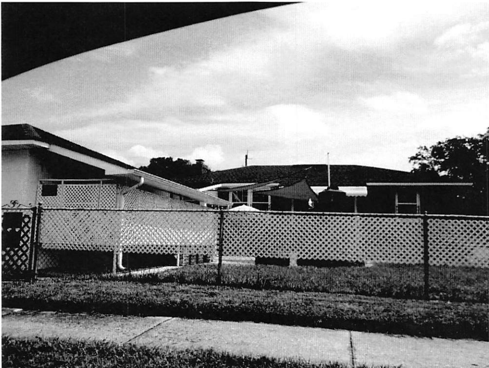
View of the residence across the street
