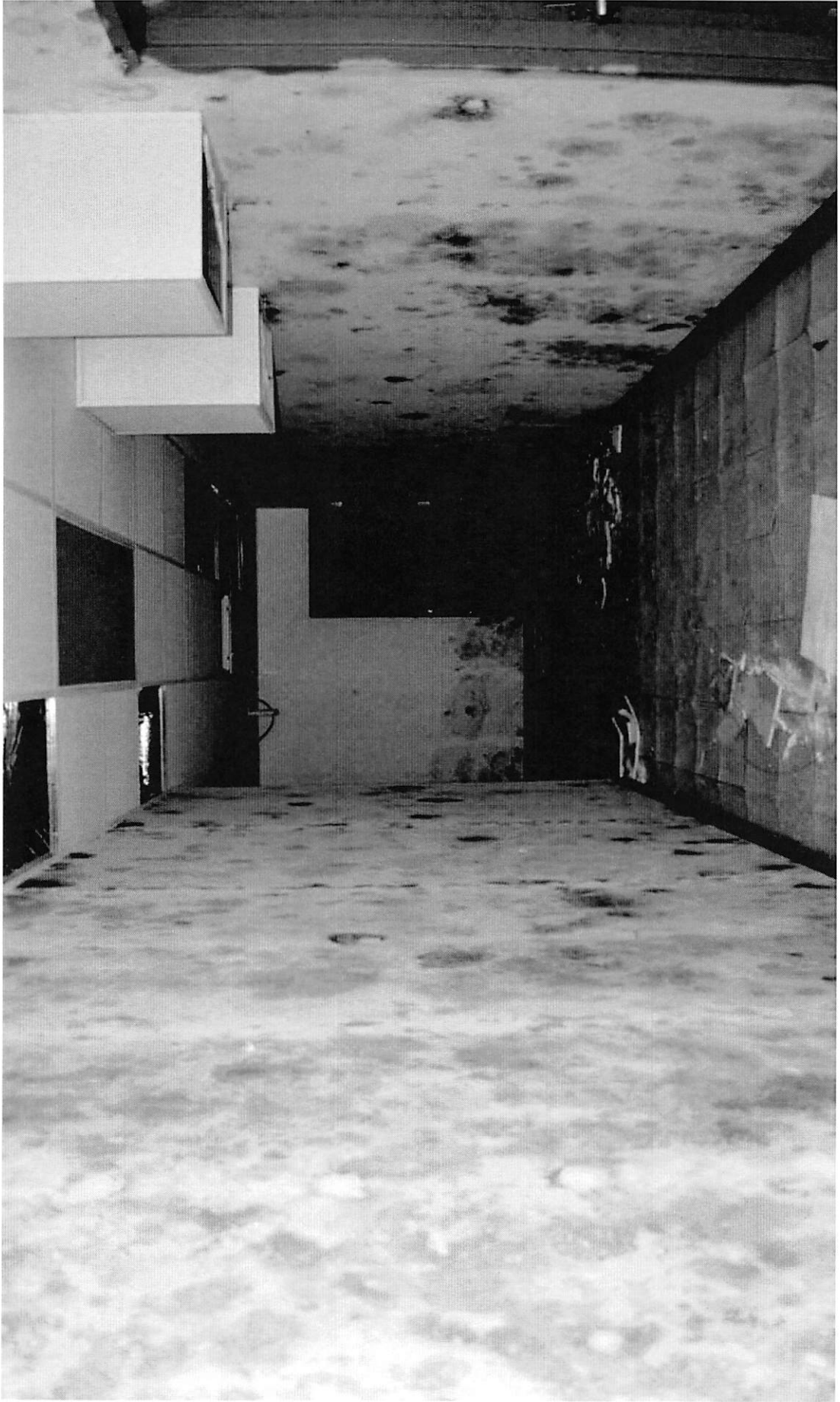
404 N. JULIA STREET, PHOTO NO. 23 HALL FACING EA ST
