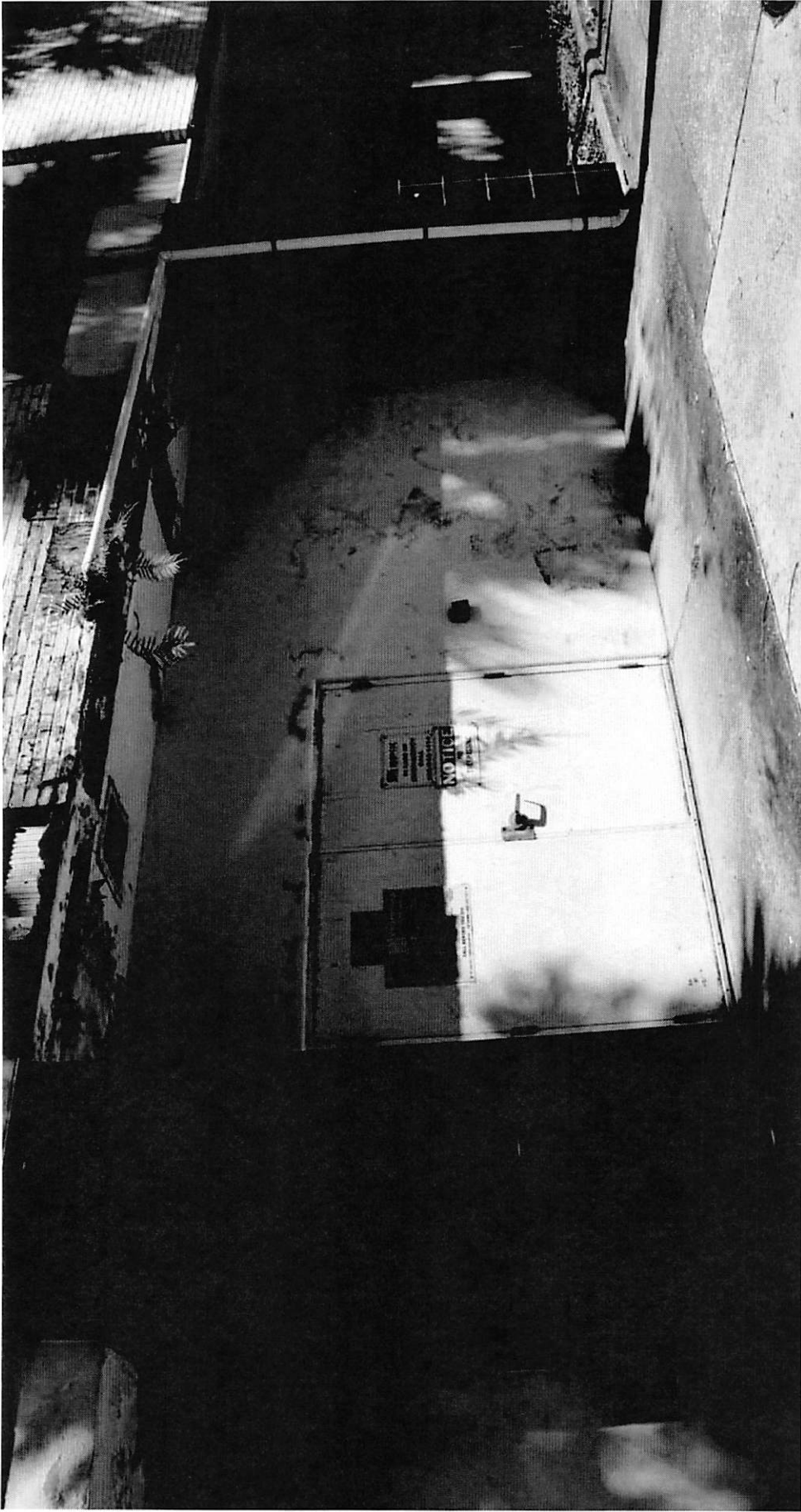
404 N. JULIA STREET, PHOTO NO. 7 2019 DUVAL ST ELEVATION
