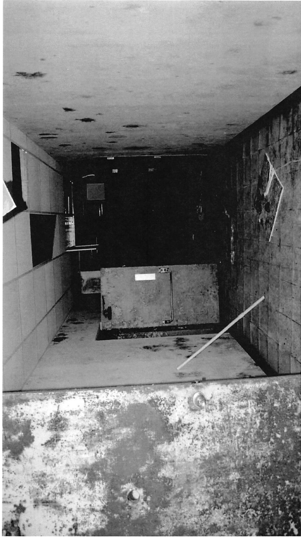
404 N. JULIA STREET, PHOTO NO. 20 DUVAL STREET ENTRANCE FACING NORTH
