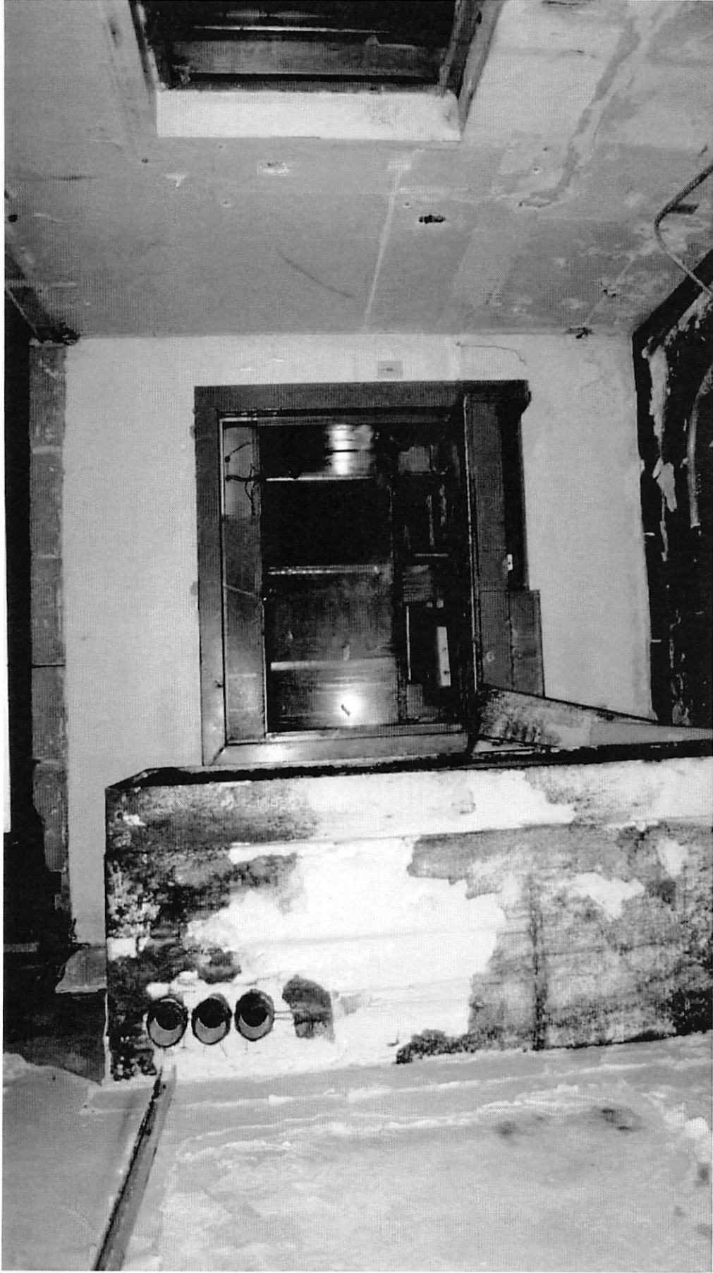
404 N. JULIA STREET, PHOTO NO. 21 DRIVE-IN TELLAR FACING WEST
