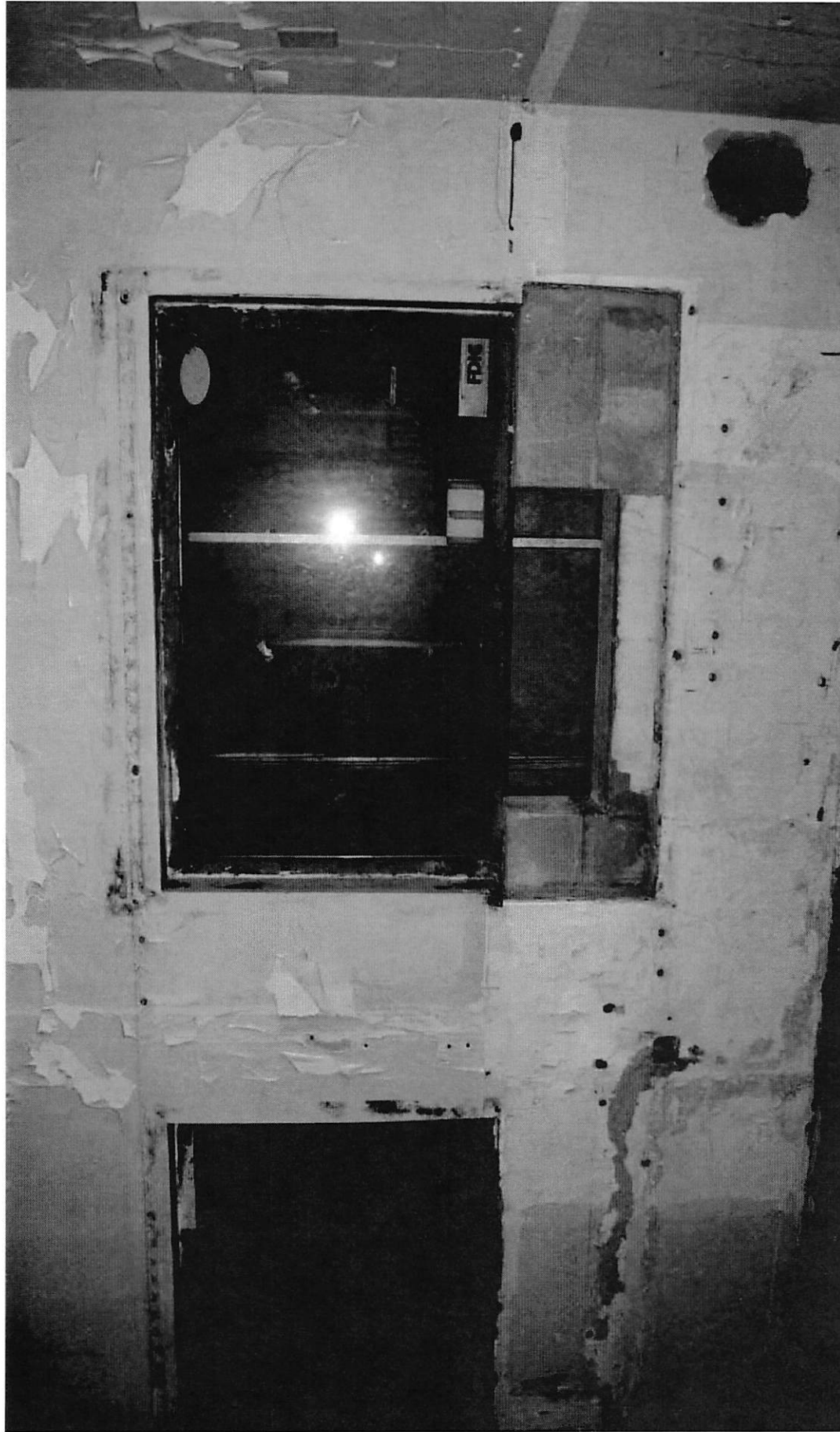
404 N. JULIA STREET, PHOTO NO. 22 DRIVE-IN TELLAR FACING WEST
