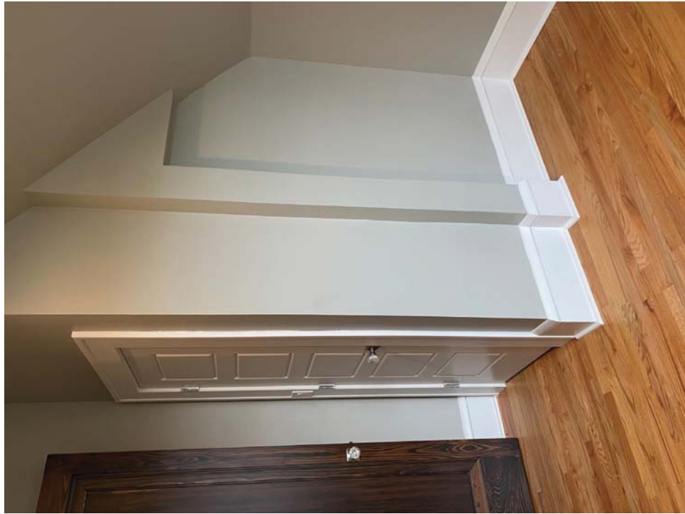
Photo 75 After (opposite view)
