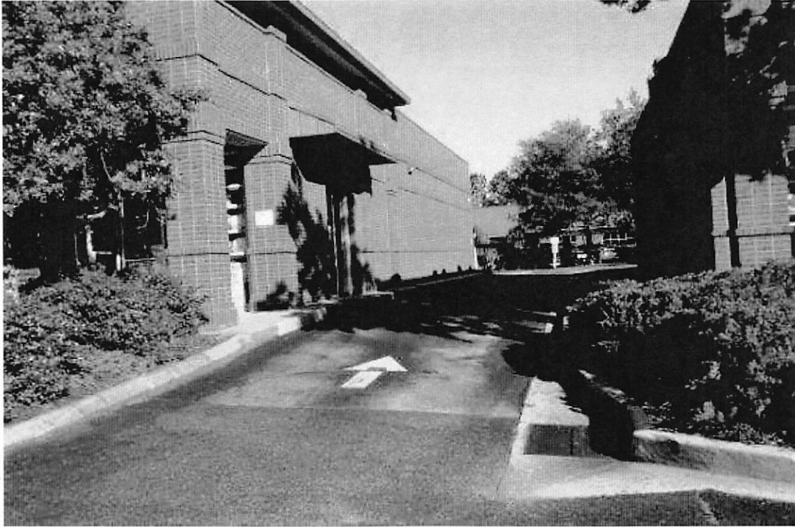
Existing drive through lane on opposite side of building
