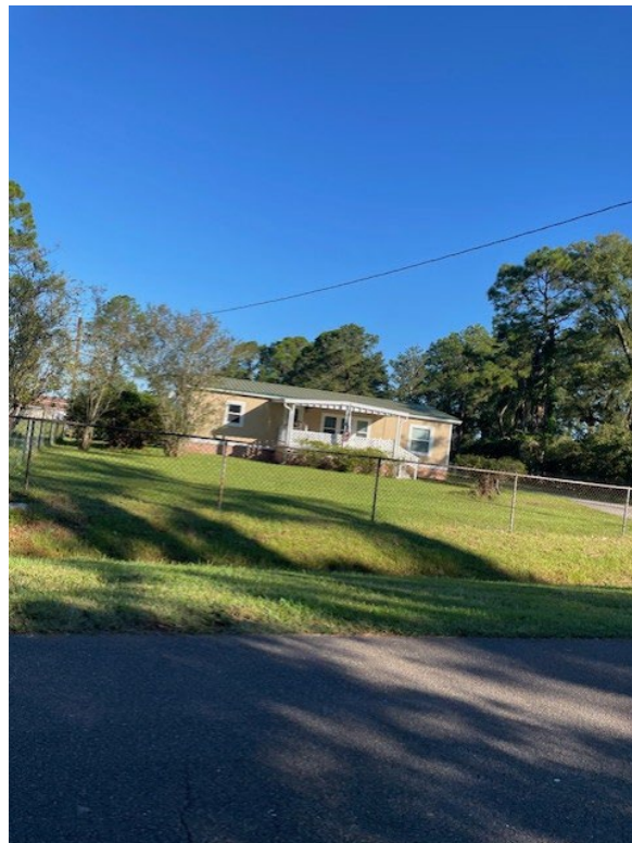
View of neighboring property, directly in front of subject property (Source: Planning Department October 2025)
