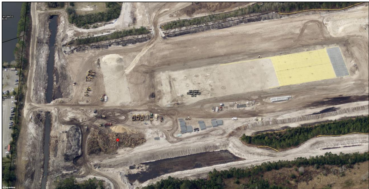
Construction of approved Warehouse Facility (CDN.3383.030)
