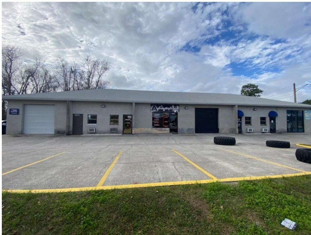
View of Existing Building 1 on site plan.
