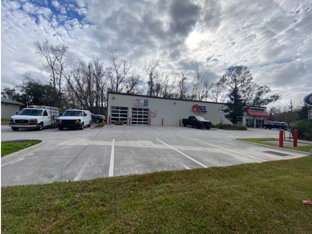
View of Existing Building 2 on site plan.
