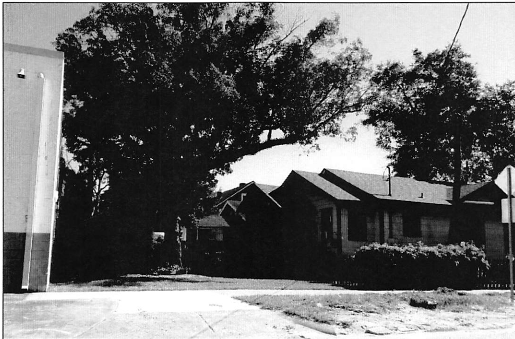
View of Property to the South
