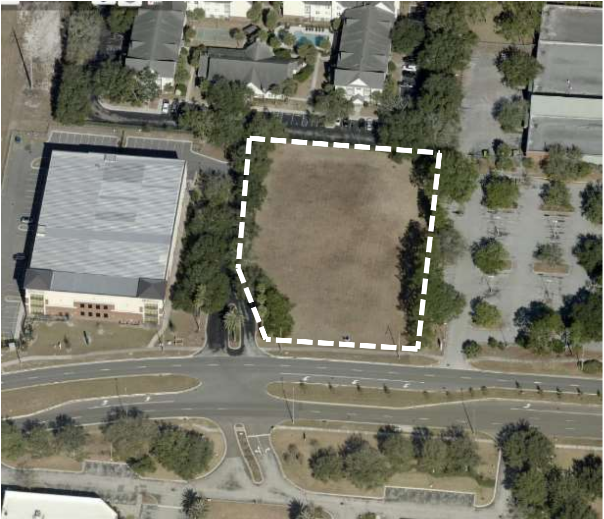
Aerial view of the subject property, facing north.
