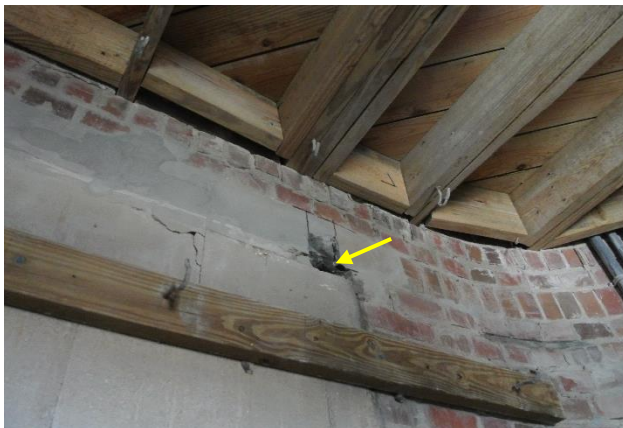
Figure 26 A small portion of the previous concrete repair was removed to expose the lintel.
