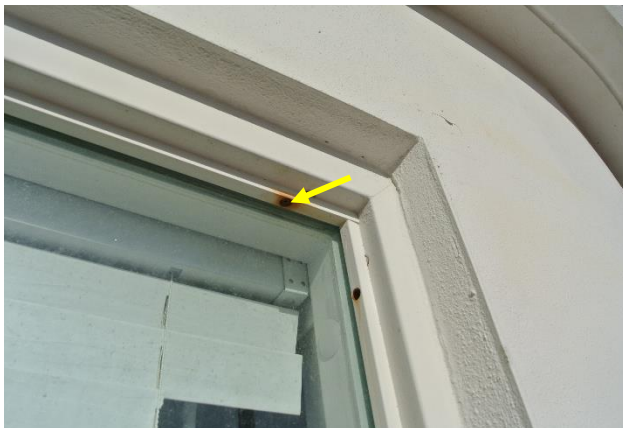
Figure 14. Window fasteners are exhibiting surface corrosion (yellow arrow).
