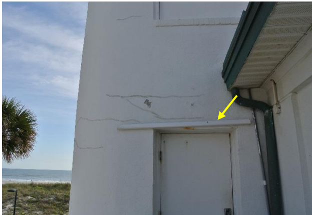
Figure 16. A gutter has been installed above a second-floor door at the watch tower (yellow arrows).
