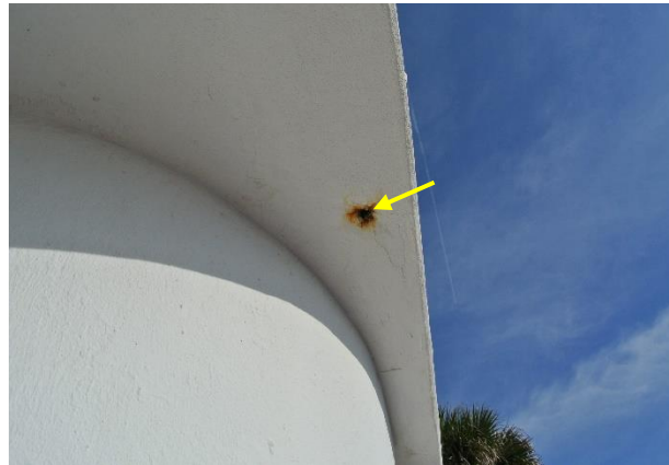
Figure 21. The drain inserts through the concrete overhang are exhibiting corrosion (yellow arrow).
