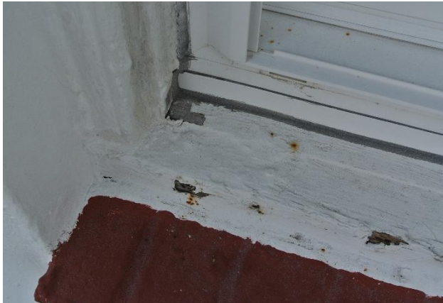
Figure 12. The wood trim around the windows is deteriorated.
