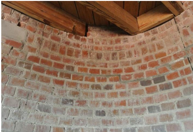
Figure 8. The interior brick wythe is exposed showing header units exclusively at the radiused corners.
