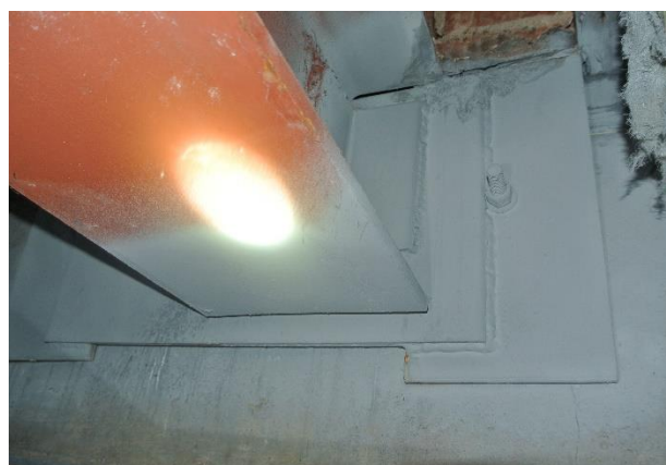
Figure 23. The new beam is welded to a plate that is welded to plates anchored into the wall.
