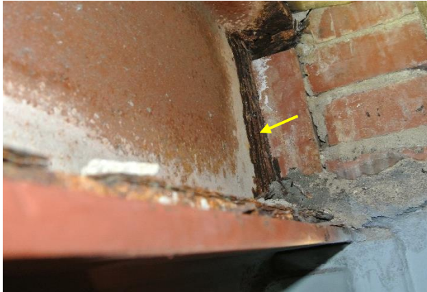
Figure 24 The existing beam is severely corroded (yellow arrow) near the exterior wall.
