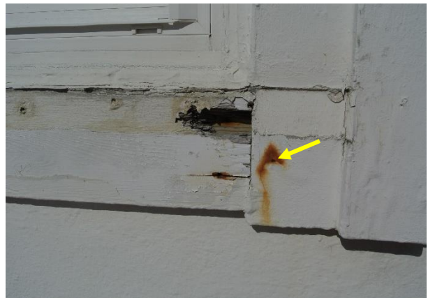
Figure 13. The wood trim around the windows is deteriorated. Corrosion staining from fasteners (yellow arrows) is also apparent.
