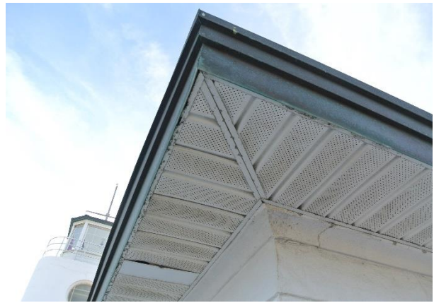
Figure 17. The eave soffit is vented around the perimeter of the two-story structure.
