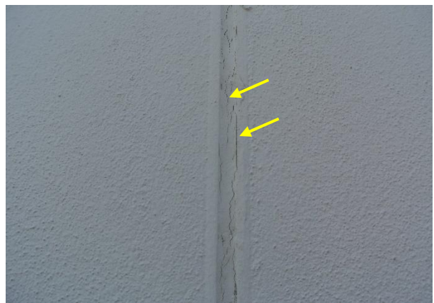
Figure 19. Sealant is experiencing adhesive and cohesive failures (yellow arrows).
