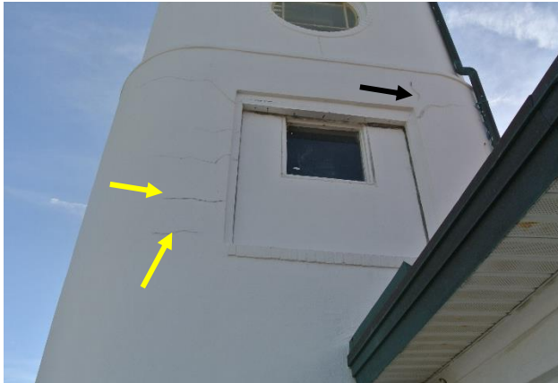
Figure 6. Radial cracks (yellow arrows) and diagonal cracks (black arrow) emanate from the window openings.
