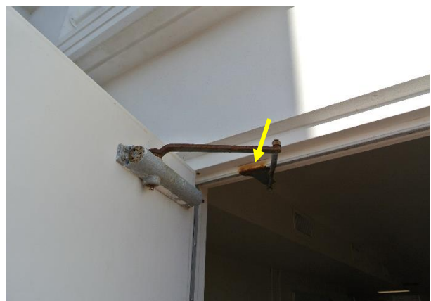
Figure 15. Door hardware throughout the facility is showing varying degrees of corrosion (yellow arrow).
