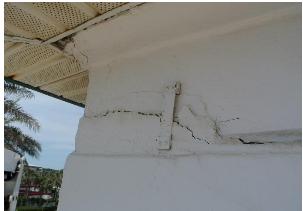
Figure 3. A sizeable crack with discernable displacement exists at the southeast corner.
