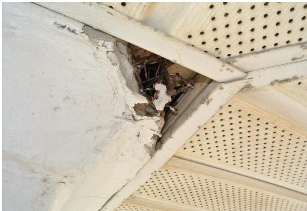
Figure 4. A small piece of ornamental stucco was loose and removed at the southeast corner.
