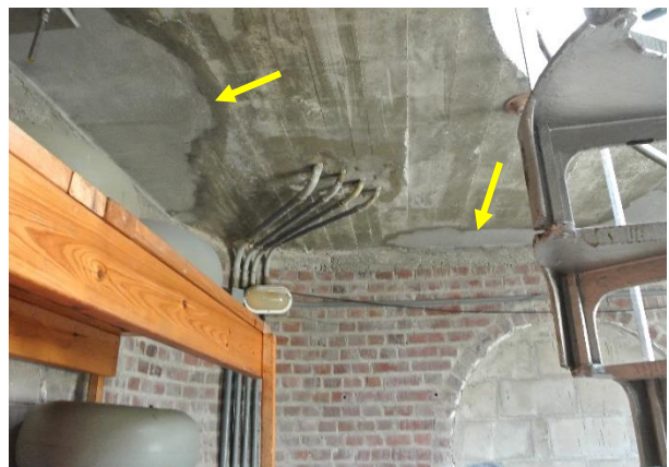
Figure 9. Previous repairs to the concrete floor slab and window headers were noted (yellow arrows).
