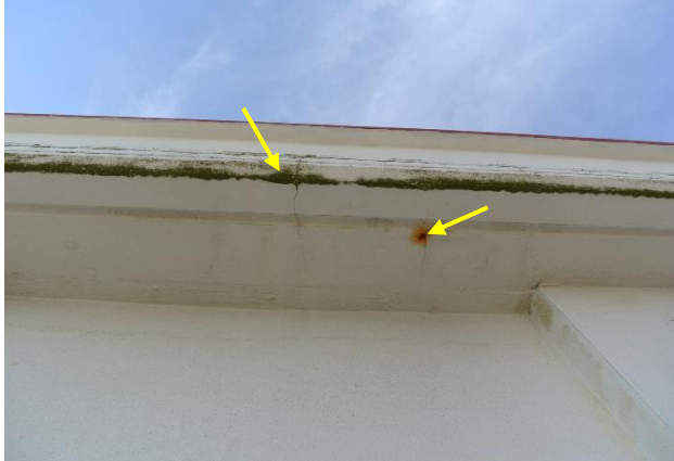
Figure 20. Biological growth, cracking, corrosion staining (yellow arrow) is present along the north facade of the addition.
