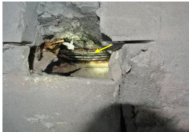
Figure 27. The steel lintel is heavily corroded similar to the steel beam in Figure 25.
