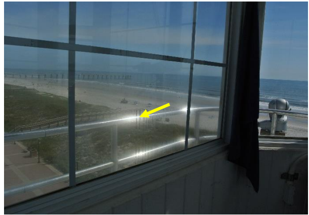
Figure 11. An IGU in the observation deck enclosure has failed. Note the condensation within the unit (yellow arrow).
