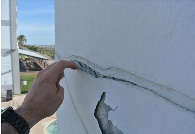
Figure 2. The coating on the stucco is peeling. The underlying stucco is cracked and delaminated.
