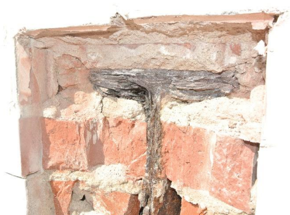
Figure 25. The end of the existing beam is thoroughly corroded where it is embedded into the brick masonry.
