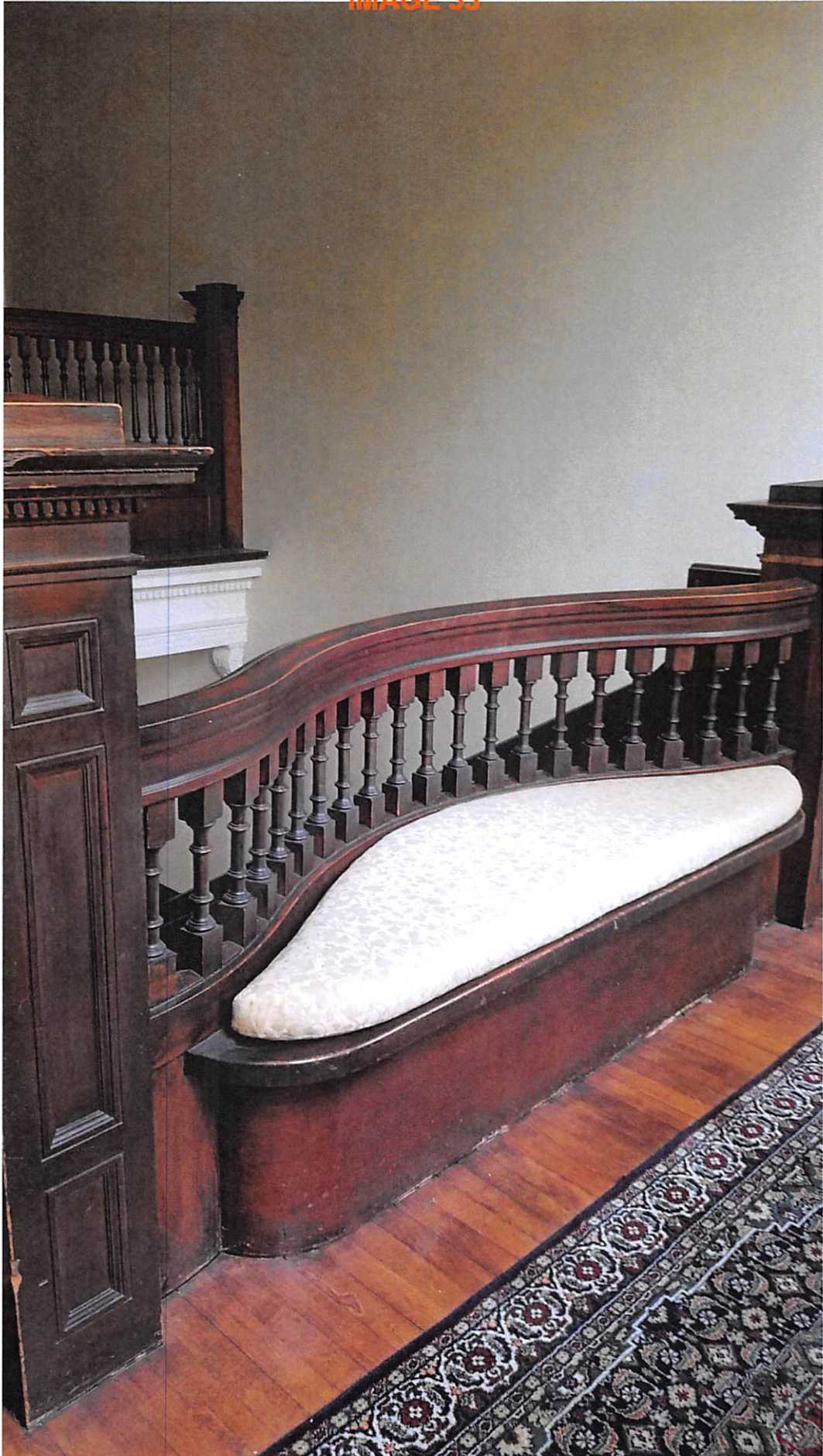
Seat at second floor landing of grand stair
