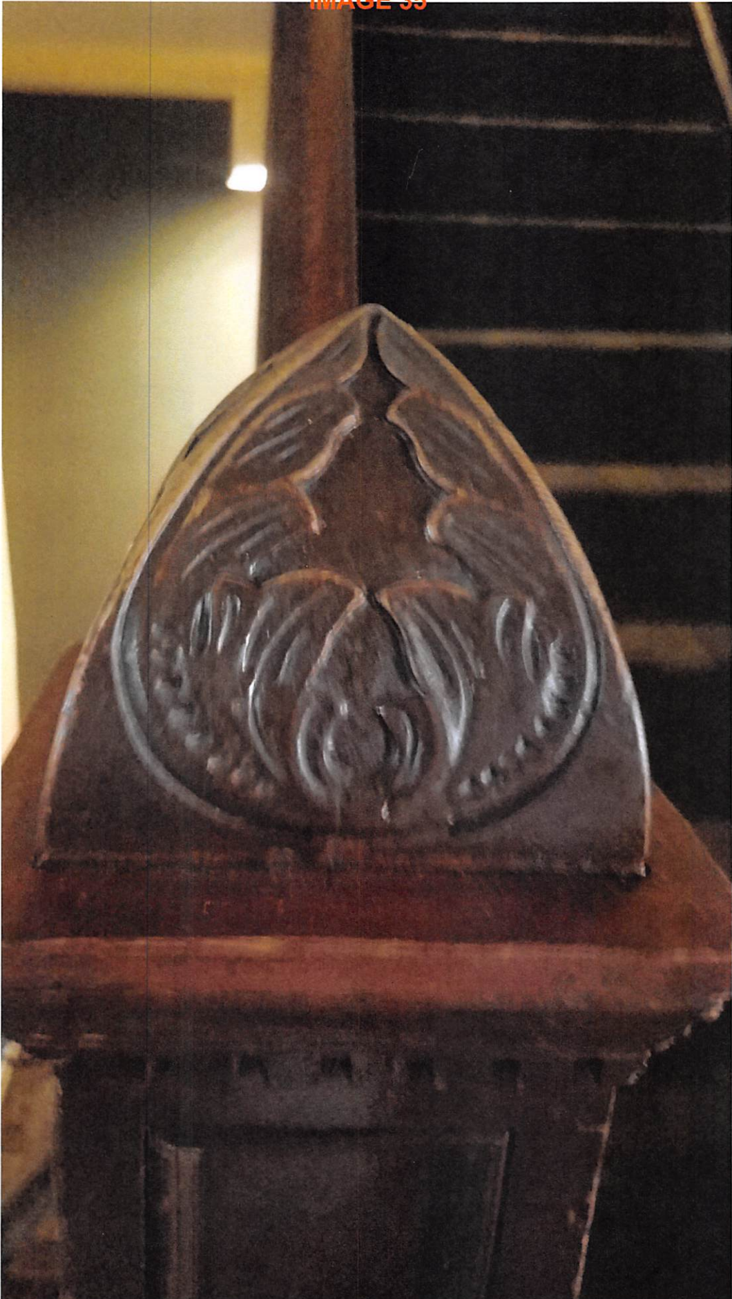
Close-up detail of servant stair newel post
