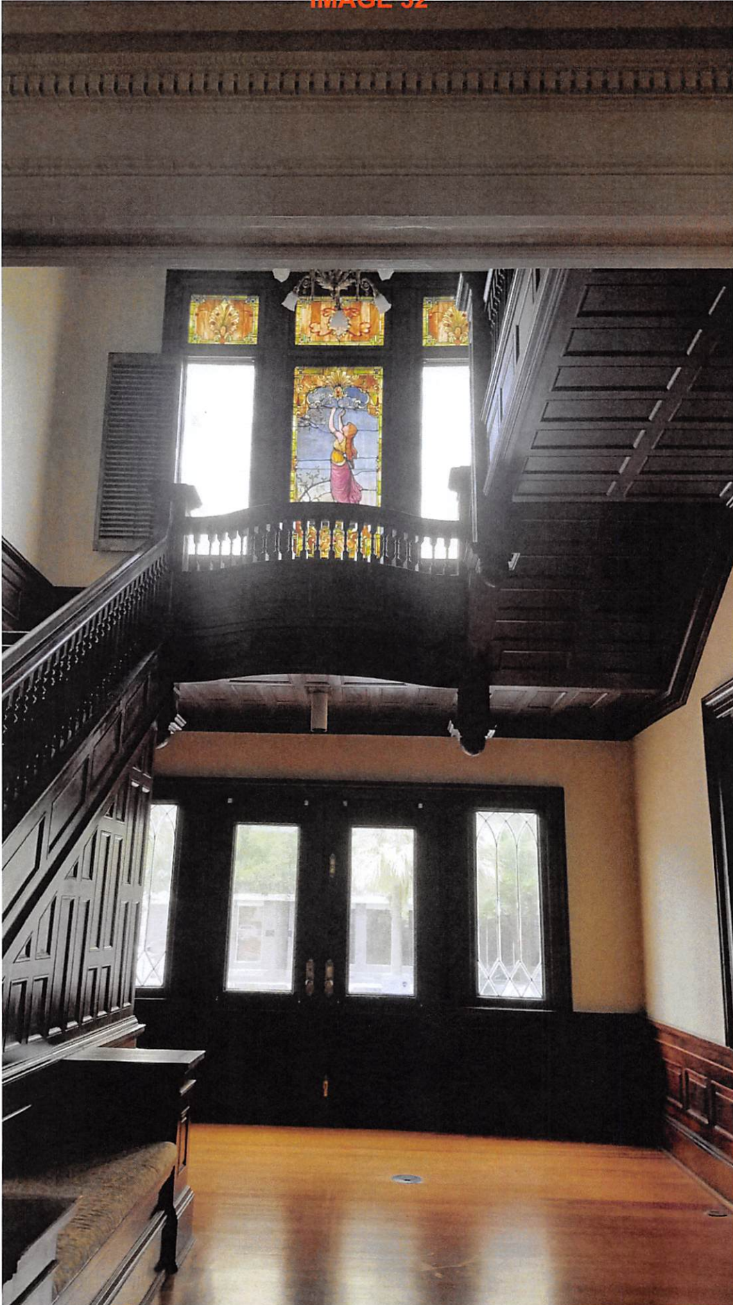
Photograph looking north at stair glass and carriage entry at grand stair
