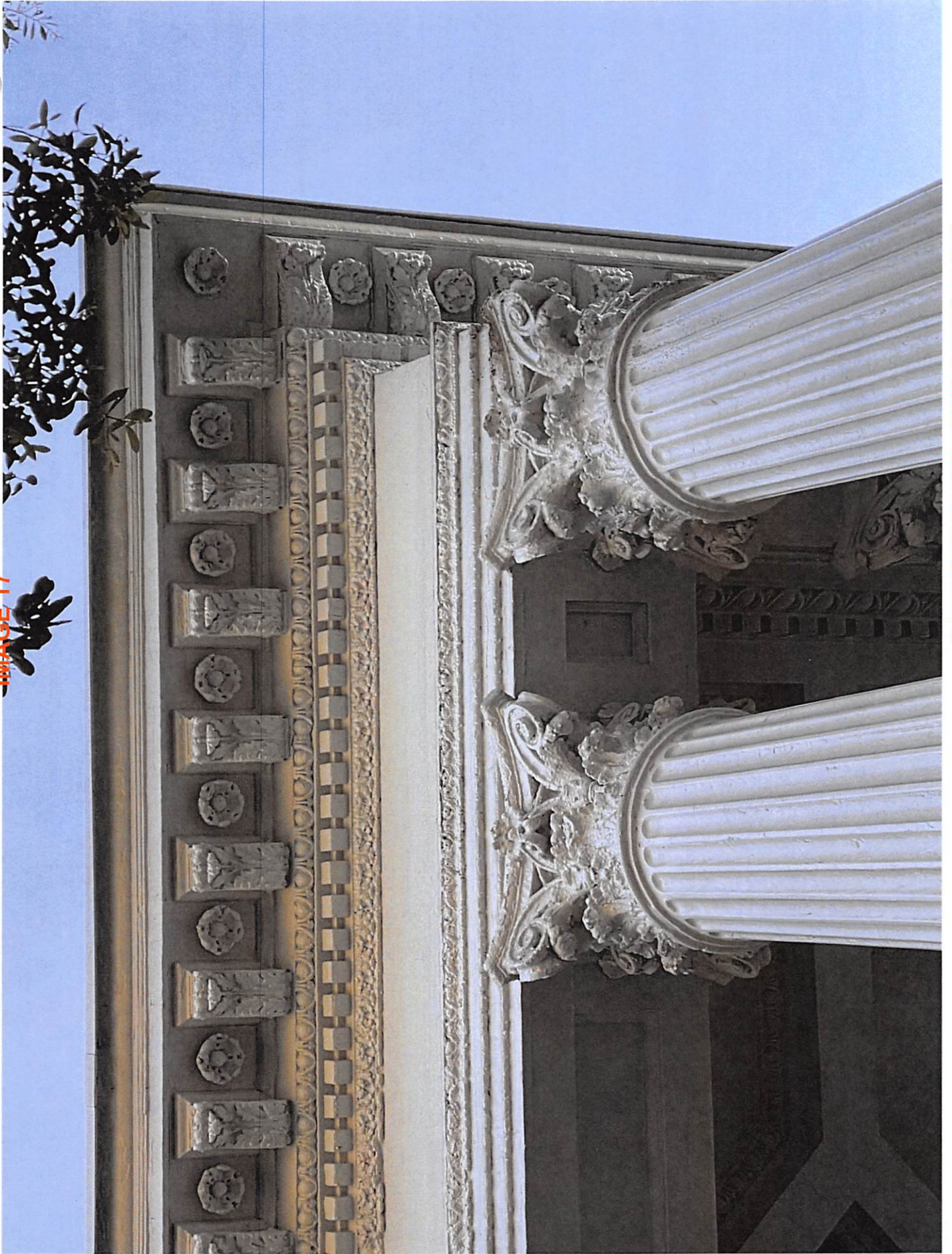
Close-up of column capitals and decorative moldings at roof
