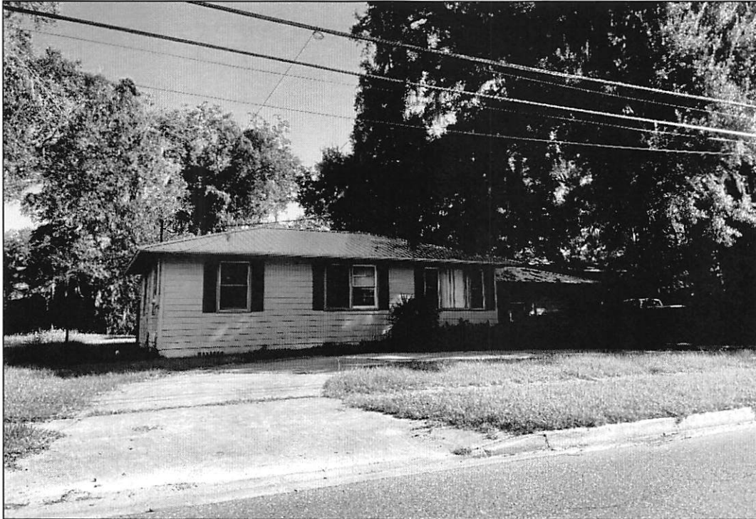
Property to the East
