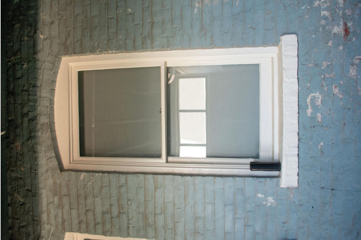
082 of 148: Interior Room 114, photographer facing west.
