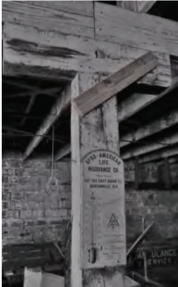
Figure 19: 2019 photograph of second floor , cassette factory support post.
