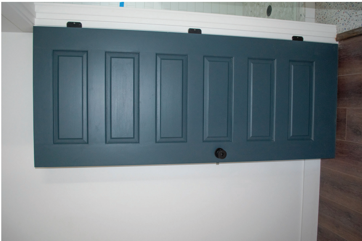
100 of 148: Interior, room 205, detail of compatible new door, photographer facing south.
