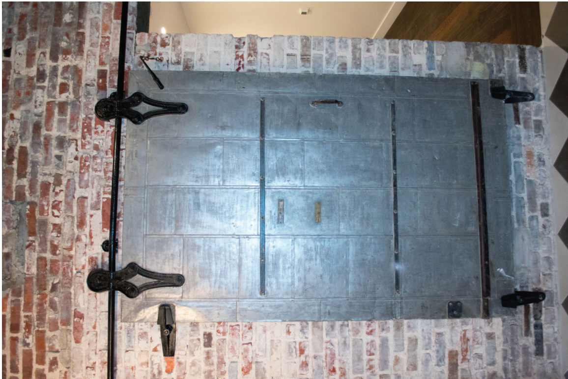
051 of 148: Interior, Room 100, photographer facing northeast.
