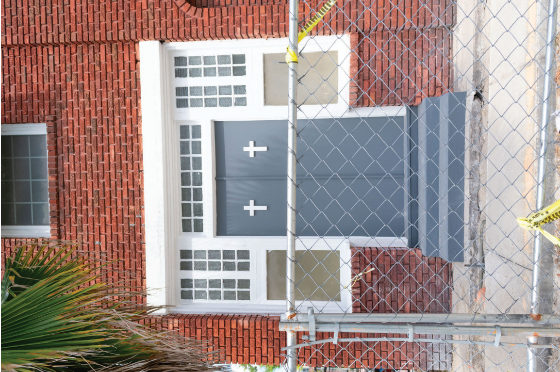
018 of 148: Exterior detail, chapel entrance, south (front) elevation, photographer facing north.
