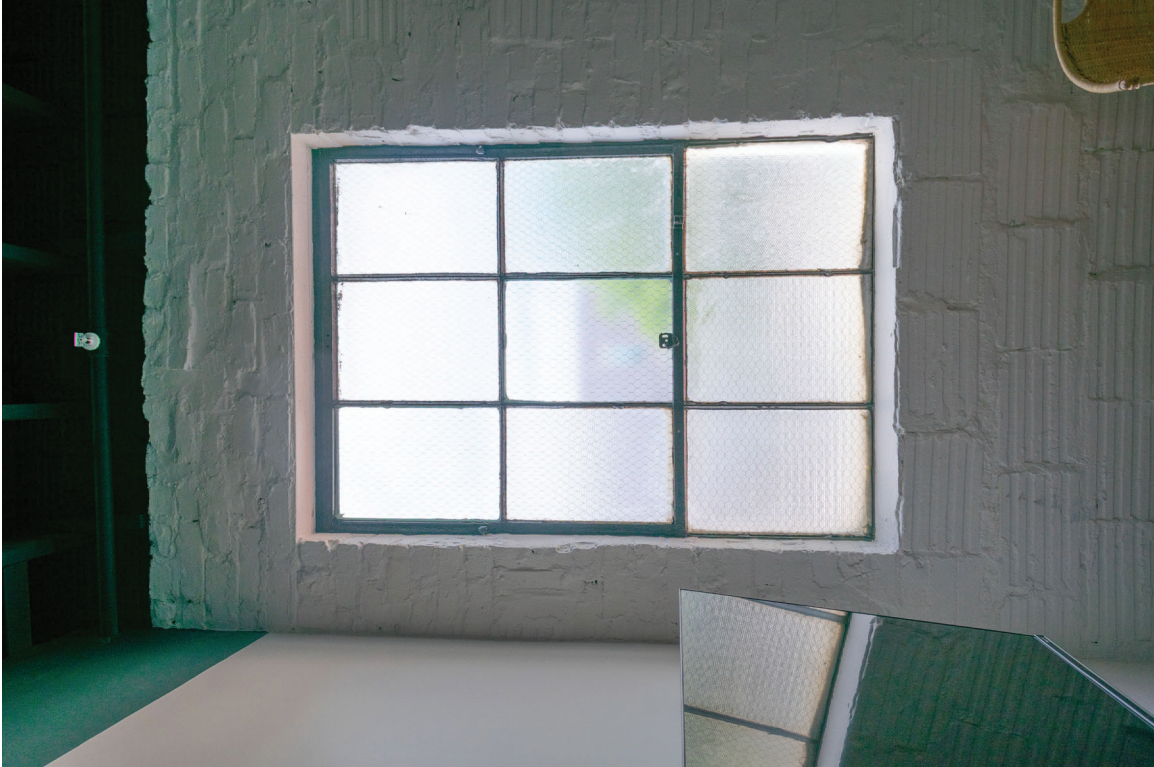
098 of 148: Interior, Room 204, detail of retained window, photographer facing west.
