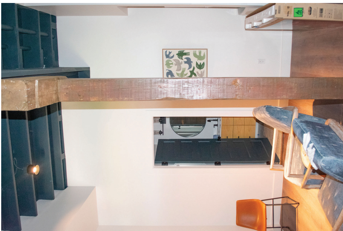
104 of 148: Interior, Room 206b, photographer facing south.
