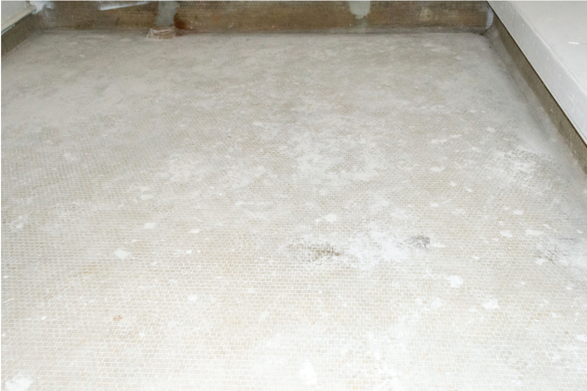
087 of 148: Interior, Room B100, retained tile floor, photographer facing east.
