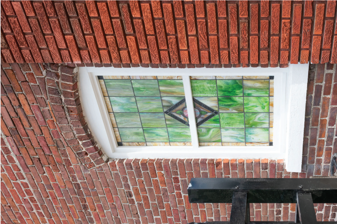
017 of 148: Exterior detail, rebuilt stained glass window, west side elevation, photographer facing northeast.
