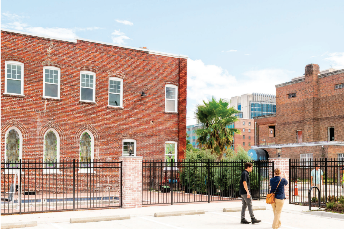
007 of 148: Exterior view, panning south to north, west side elevation; photographer facing southeast.
