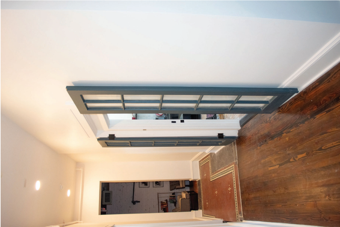
129 of 148: Interior, Room 215, photographer facing north.
