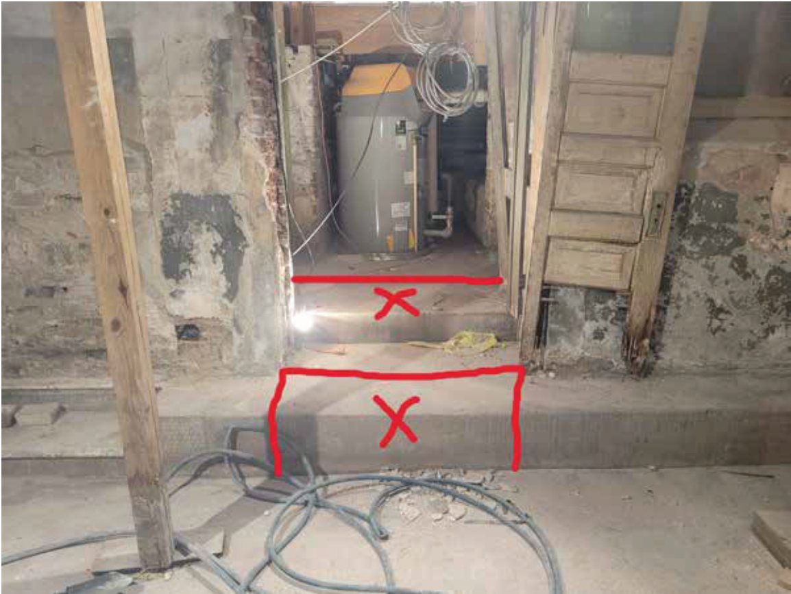
Figure A-1: These steps will be lowered to meet code. Build back will be concrete. The main tile floor will be unaltered.
