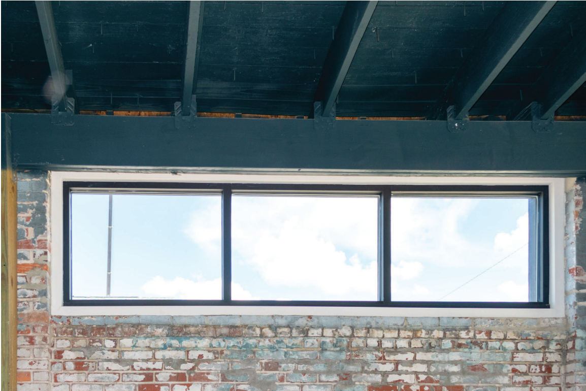
079 of 148: Interior, Room 114, photographer facing east.
