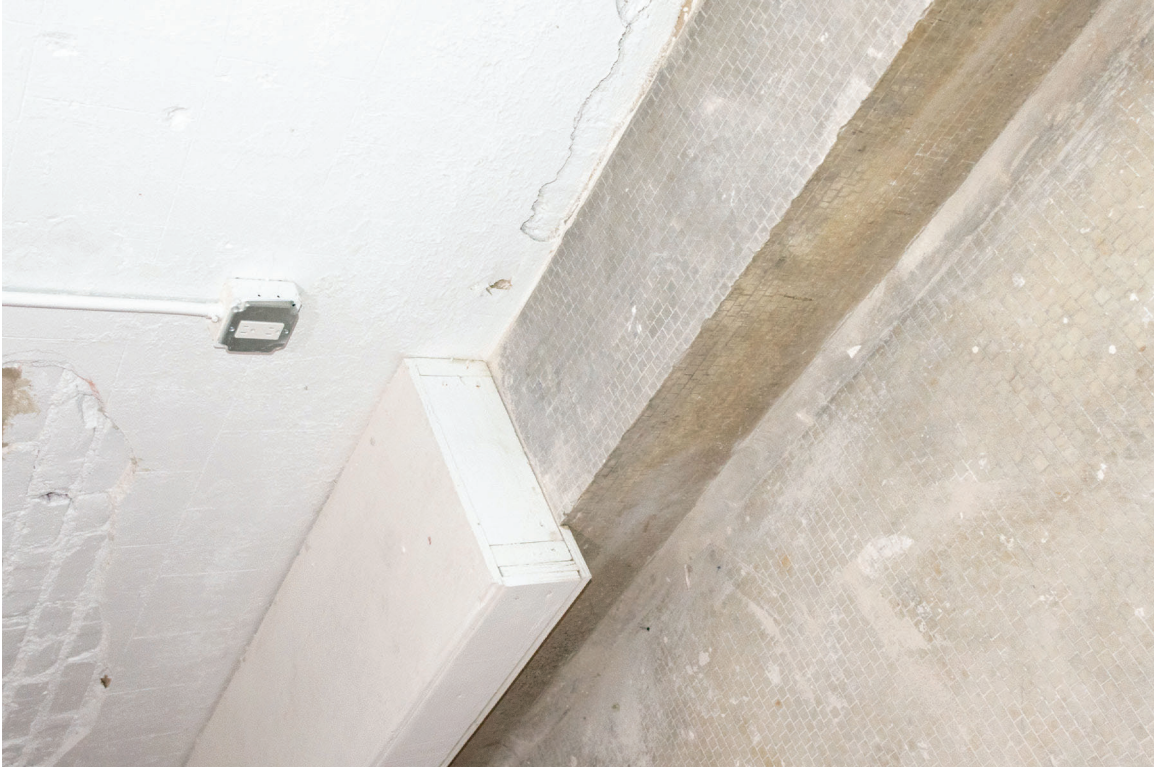
086 of 148: Interior, Room B100, photographer facing southeast.
