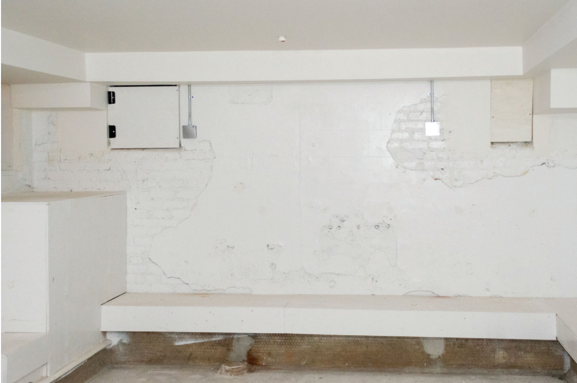
088 of 148: Interior, Room B100, photographer facing east.
