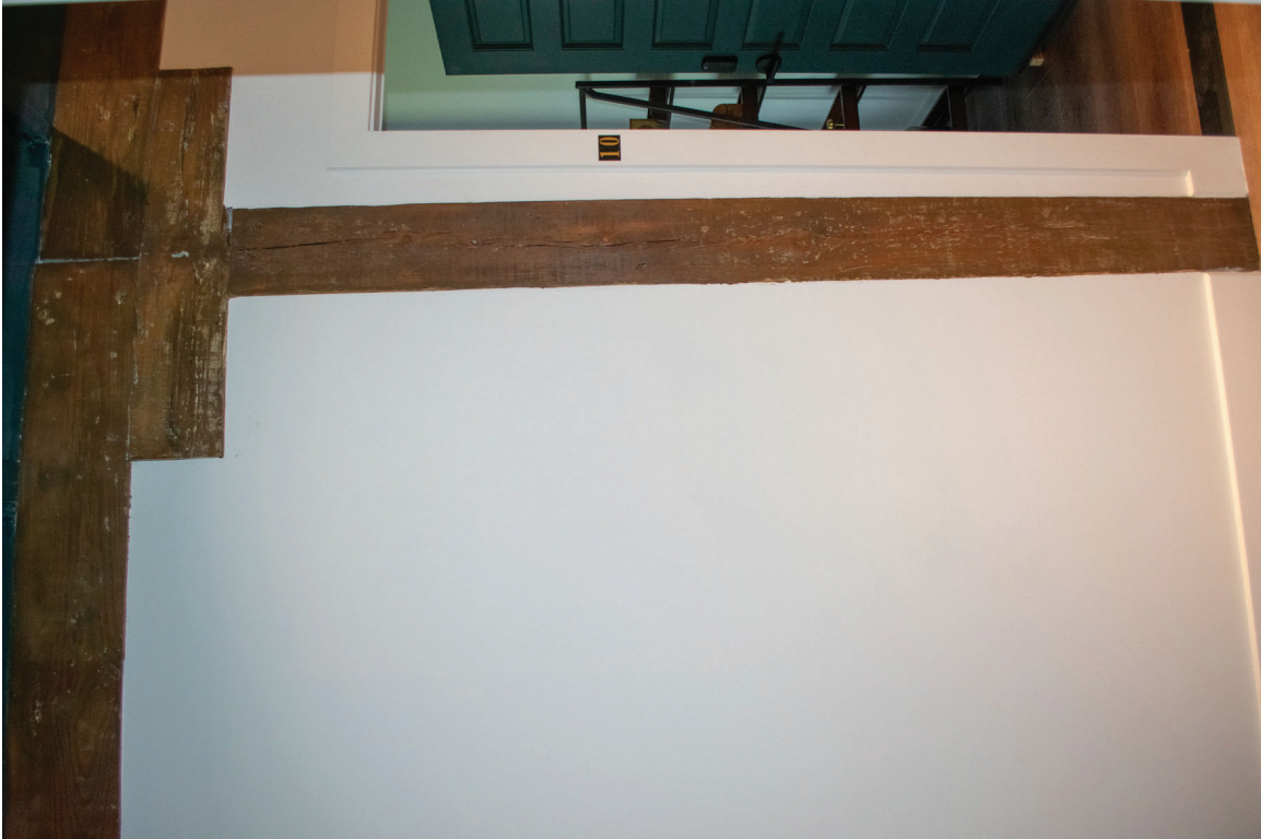
109 of 148: Interior, Room 201, detail of exposed beam, photographer facing east.
