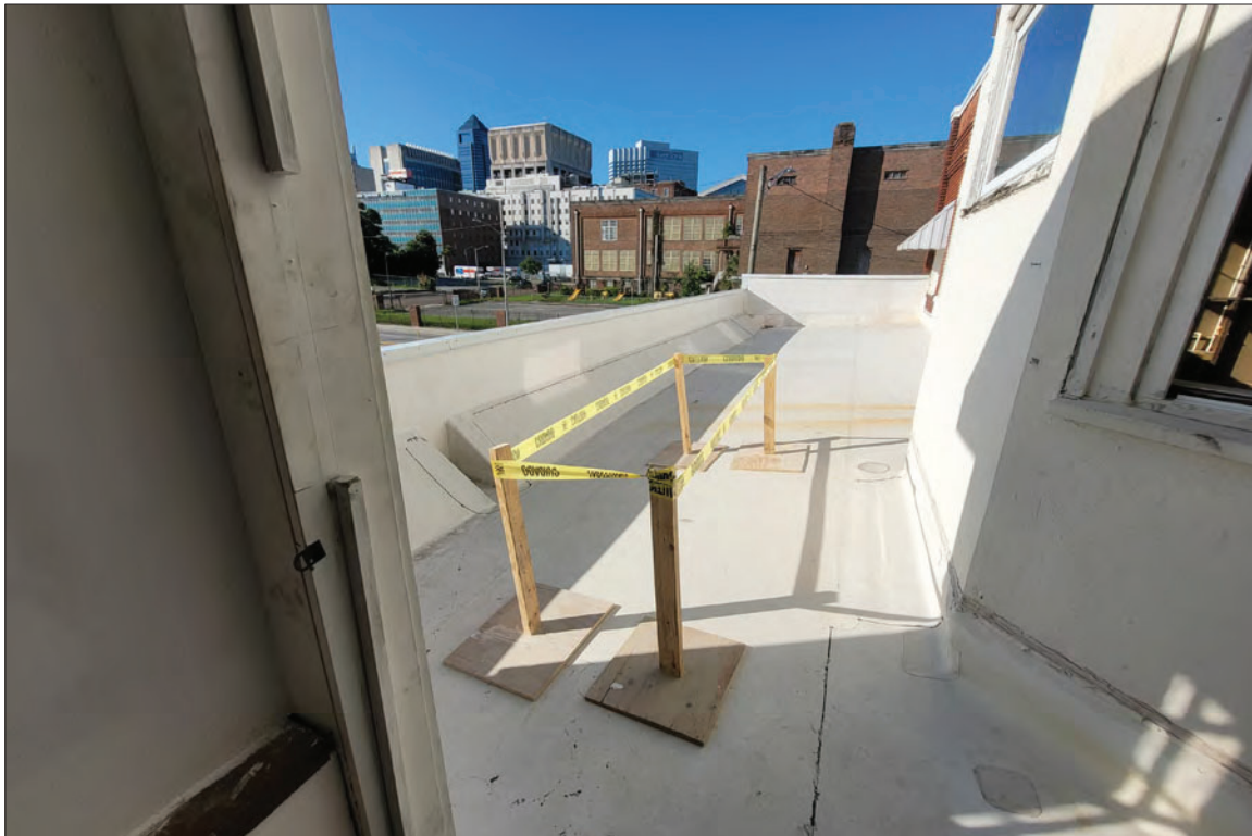
1.2l: Condenser mock up on roof, see locations A - C on Figure 1.2a; photographer facing south.
