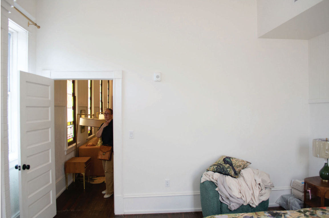
048 of 148: Interior, Room 118, photographer facing north.
