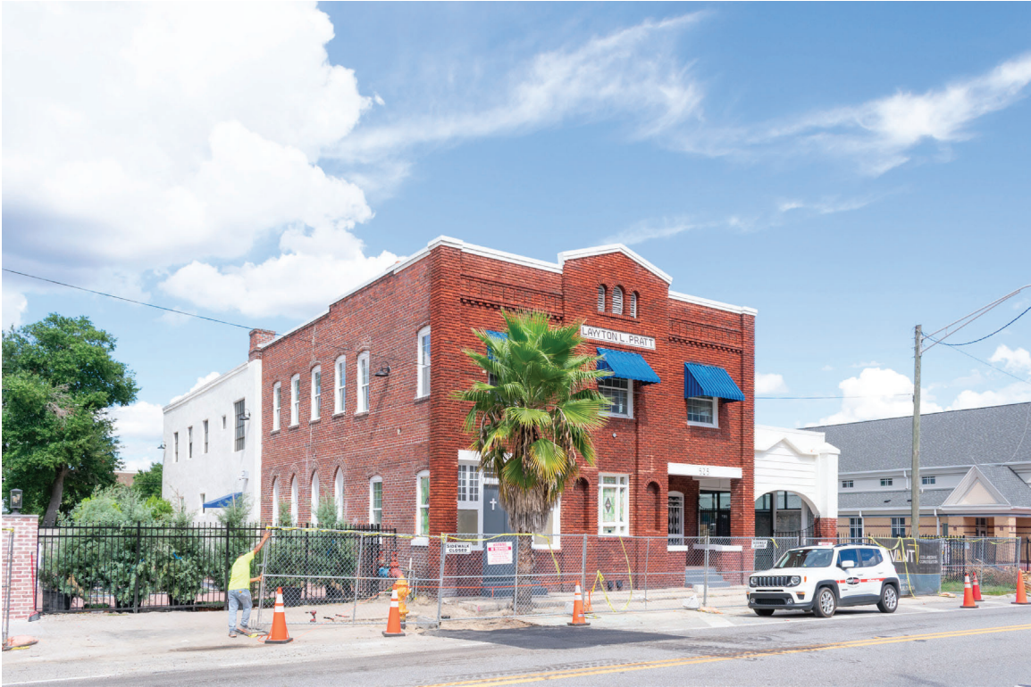
005 of 148: Exterior view, south (front) and west side elevations; photographer facing northeast.
