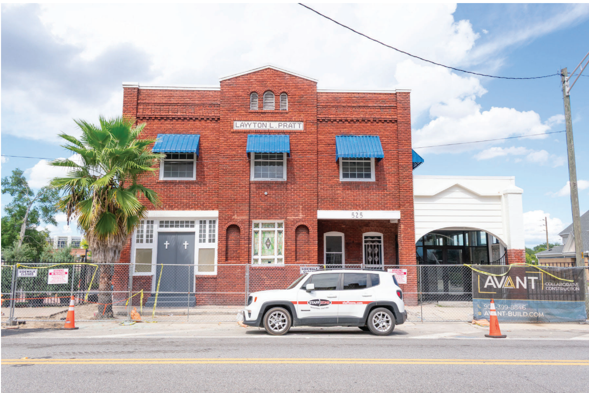
004 of 148: Exterior view, south (front) elevation; photographer facing north.
