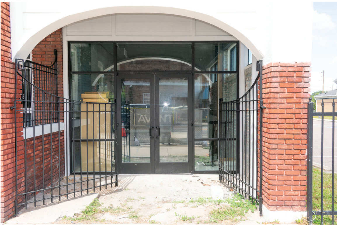
024 of 148: Exterior detail, recessed drive, photographer facing north.
