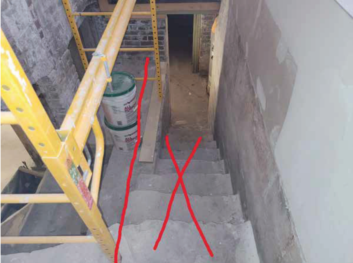
Figure A-2: The existing concrete steps to the basement will be demolished and built back to code making them approximately 12" wider. It is likely this concrete is a nonhistoric addition. Buildback will be concrete.
