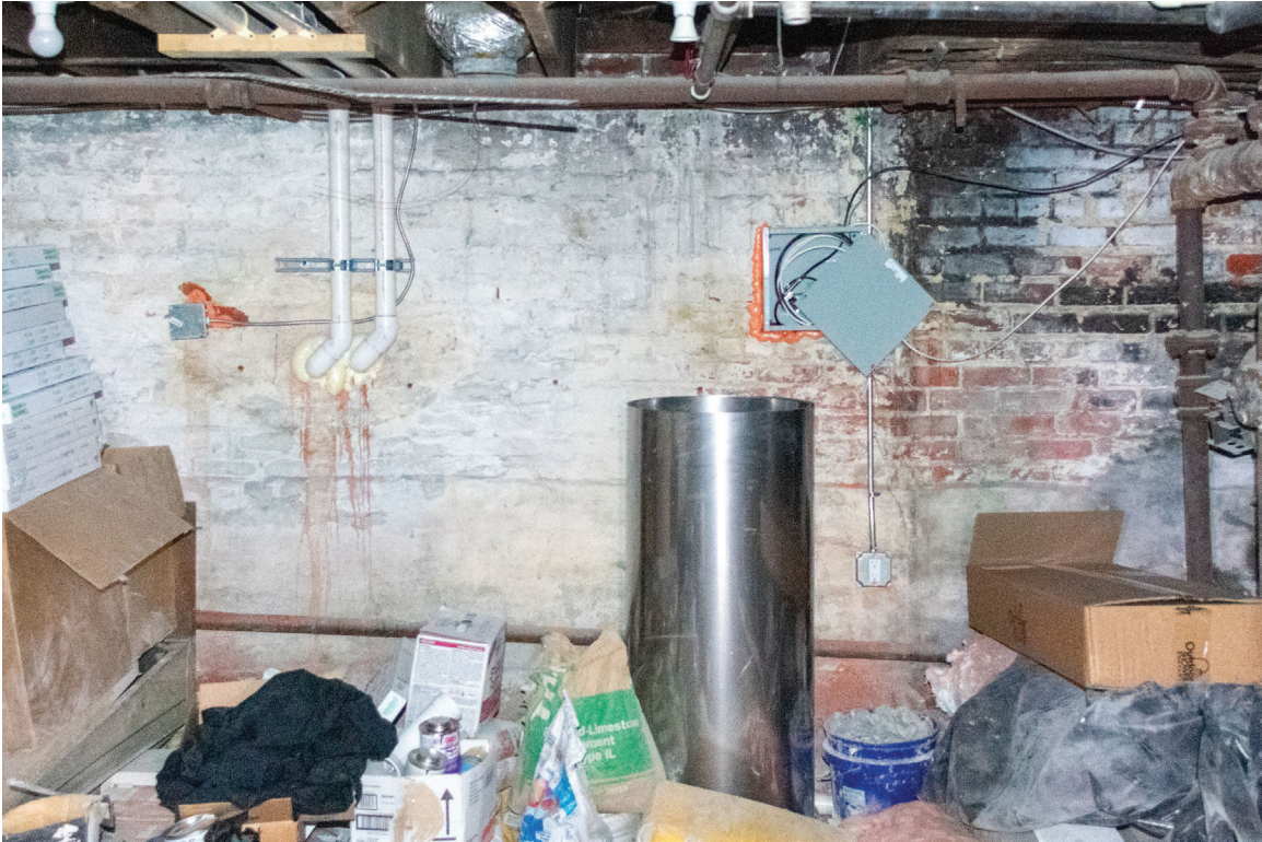
089 of 148: Interior, Room B101, photographer facing west.
