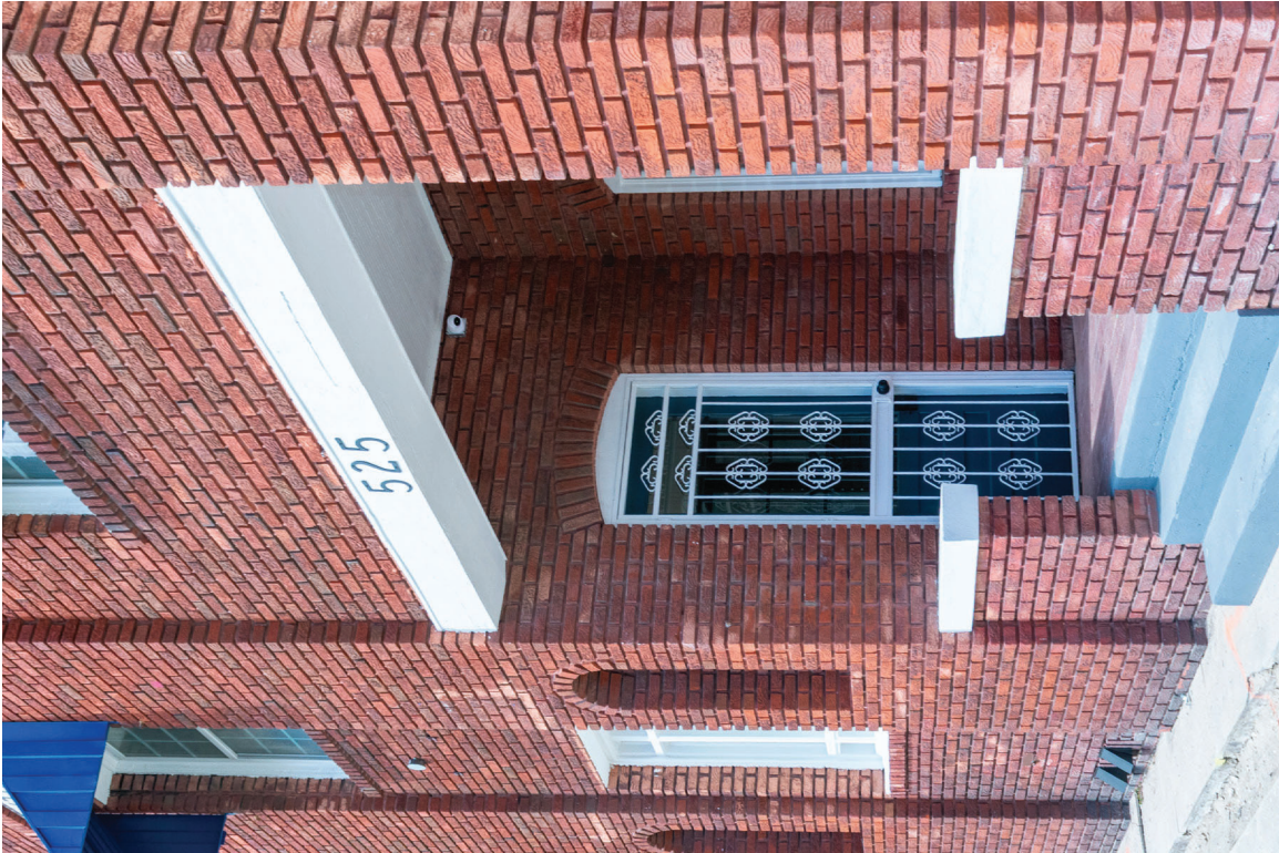
023 of 148: Exterior detail, office bay, recessed porch, photographer facing northwest.
