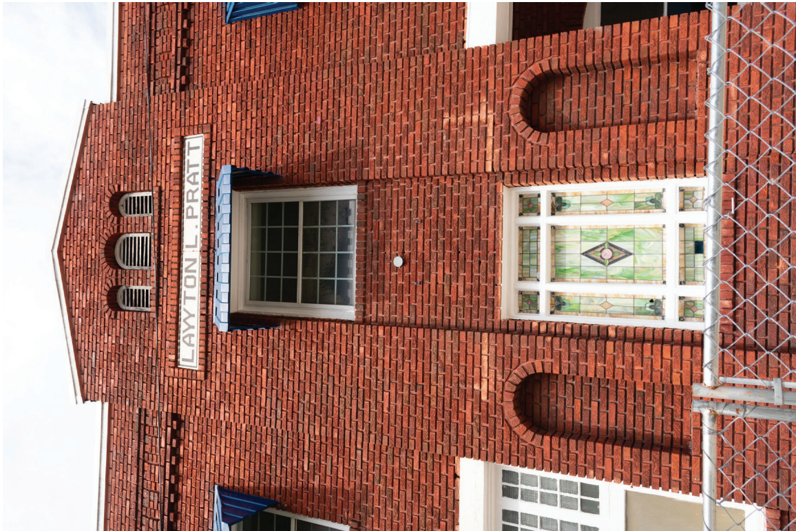
019 of 148: Exterior detail, central bay, south (front) elevation, photographer facing north.
