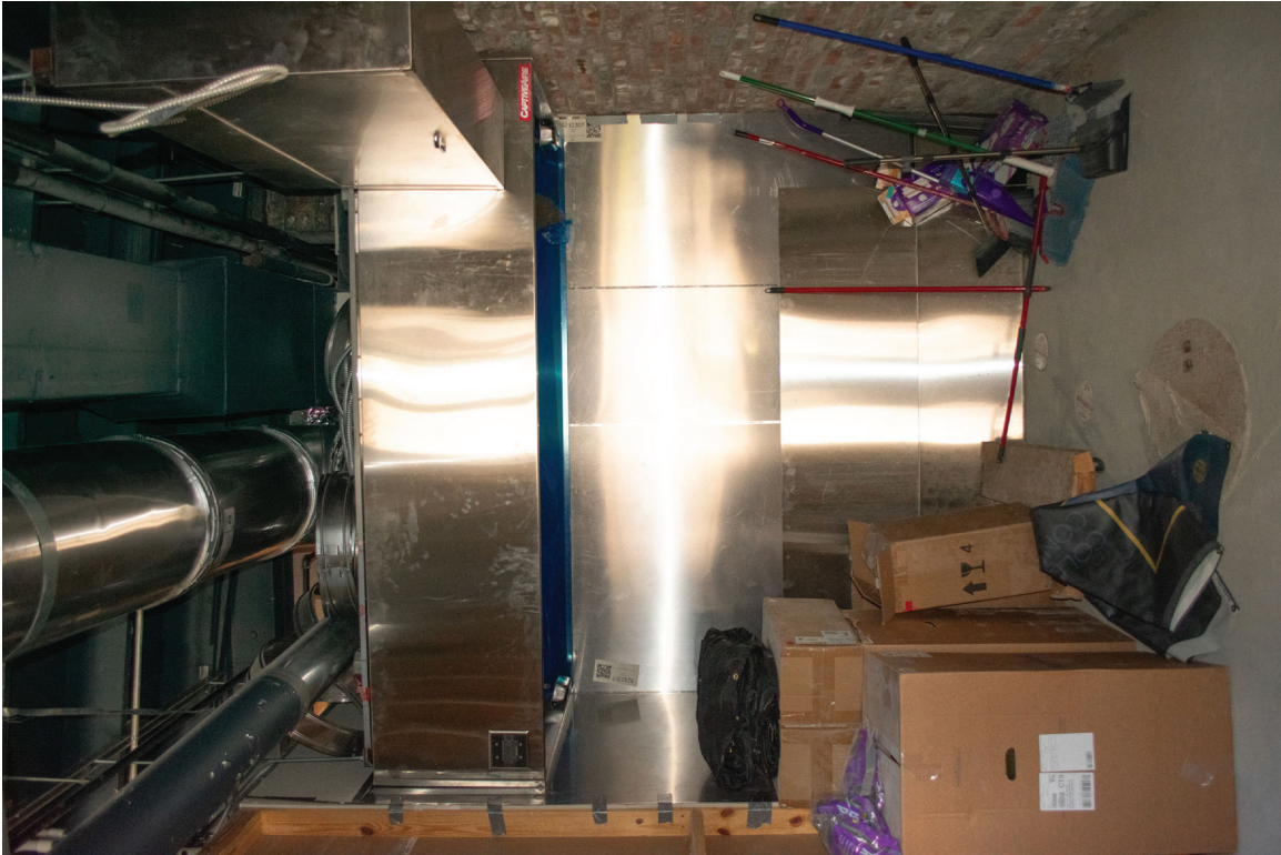
081 of 148: Interior, Room 112, photographer facing north.
