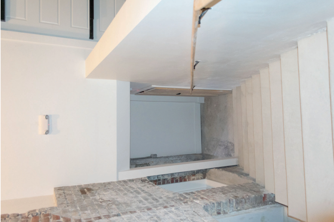
084 of 148: Interior, Room 110, photographer facing west.
