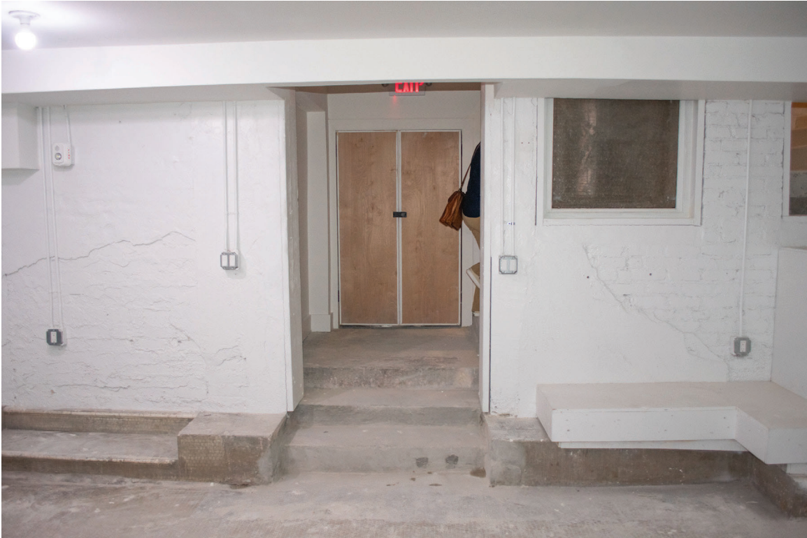
091 of 148: Interior, Room B100, photographer facing north.
