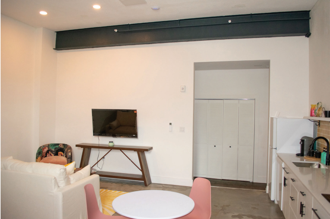
064 of 148: Interior, Room 104, photographer facing northeast.
