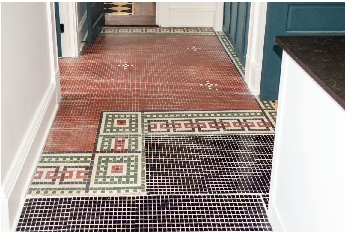
148 of 148: Interior, Room 222, detail of uncovered tile, photographer facing north.
