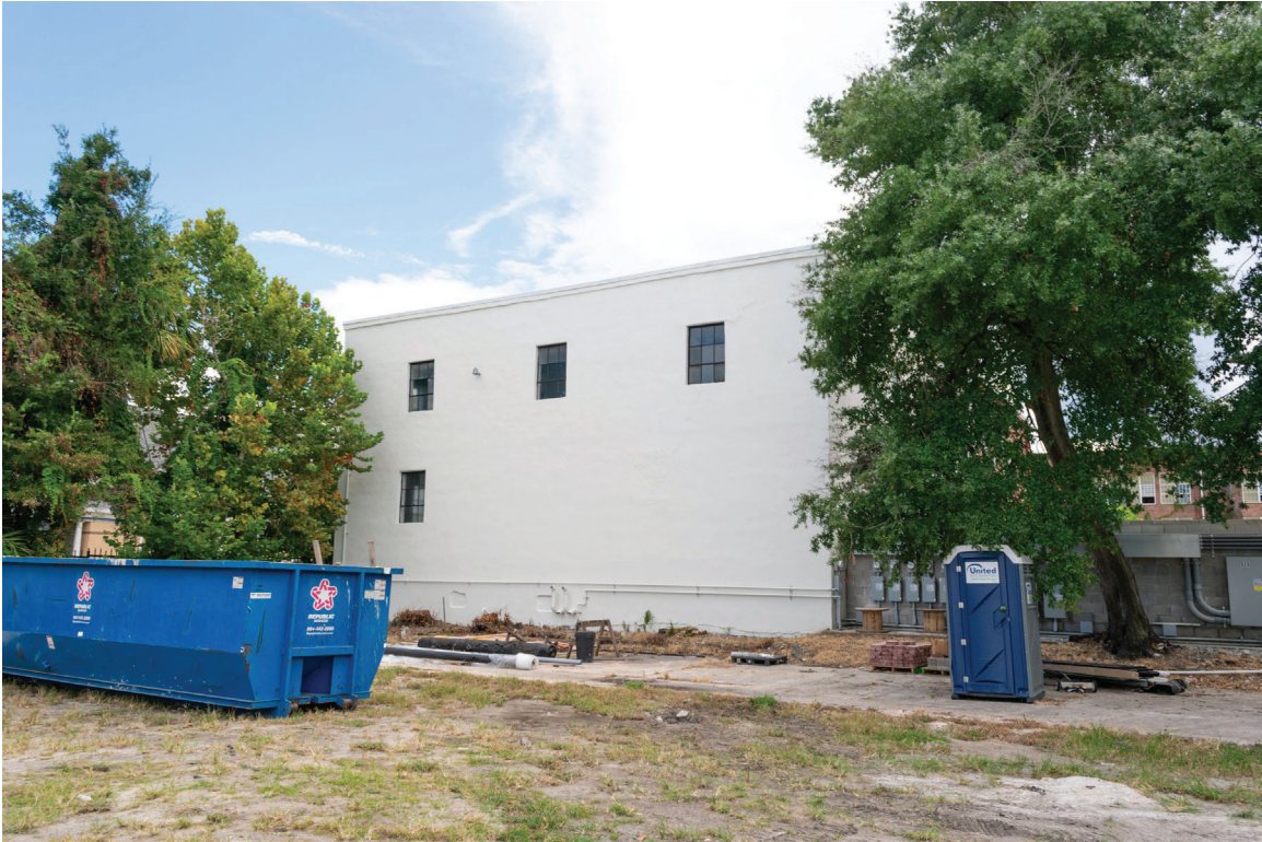
001 of 148: Exterior view, north (rear) elevation; photographer facing southeast.
