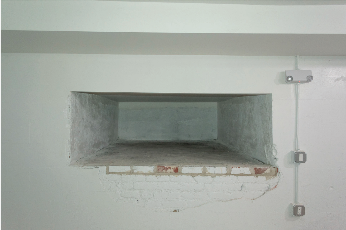
085 of 148: Interior, Room B100, photographer facing south.
