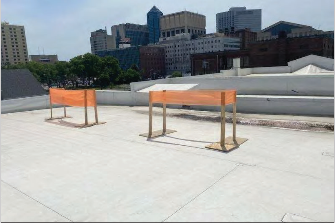
1.2b: Condenser mock up on roof, see locations A - C on Figure 1.2a; photographer facing southeast.
