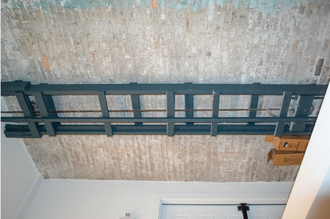
092 of 148: Interior, Room 110, photographer facing northeast.
