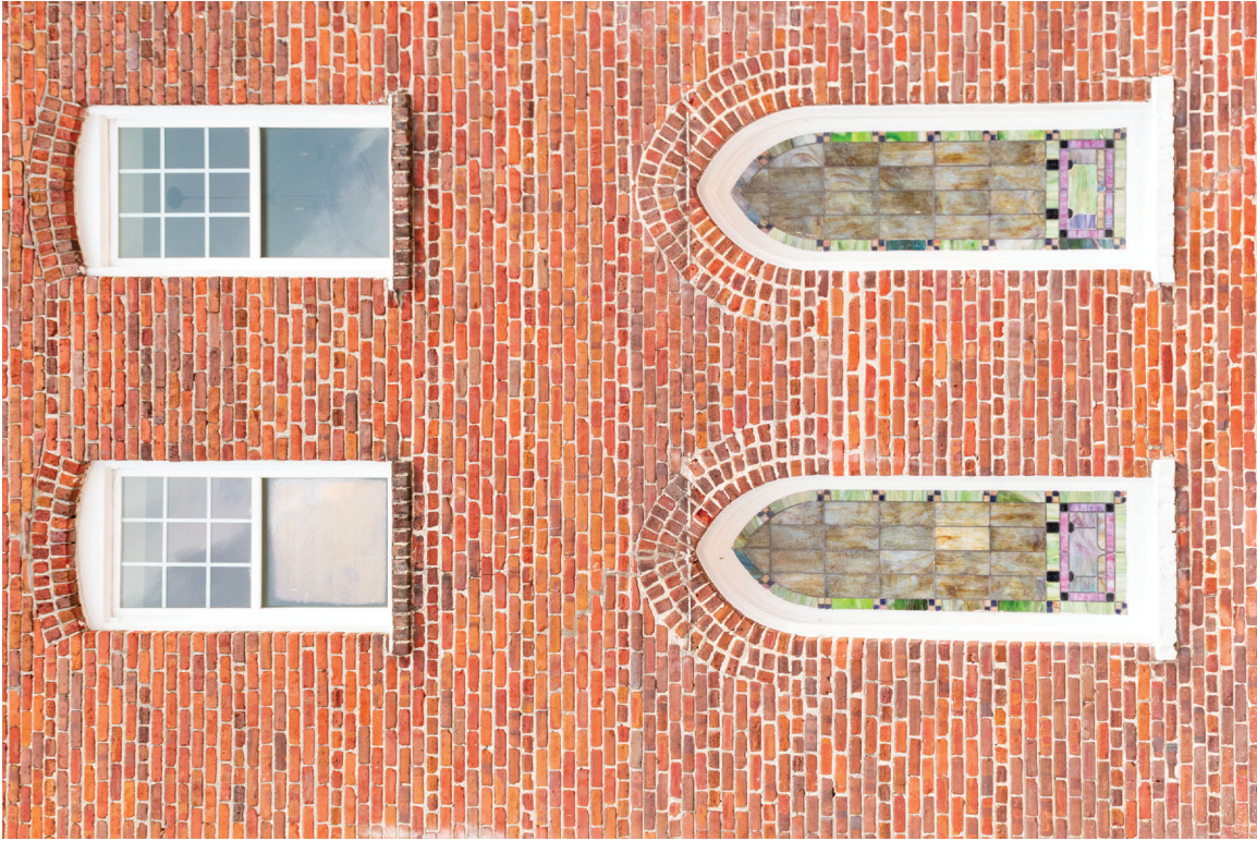
027 of 148: Exterior detail, chapel windows, west side elevation, photographer facing east.
