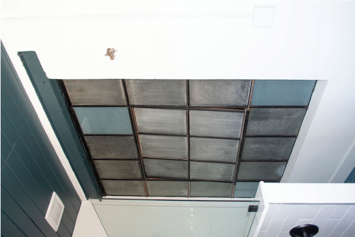
119 of 148: Interior, Room 213, detail of retained window, photographer facing northwest.
