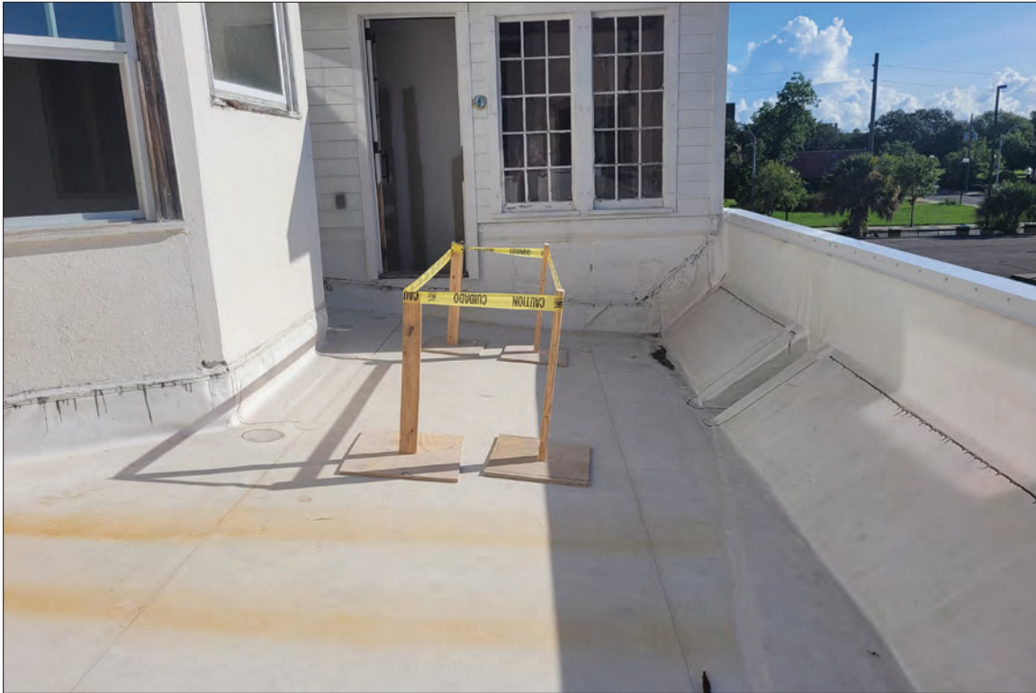
1.2k: Kitchen venting mock up on covered driveway, see locations D on Figure 1.2a; photographer facing northeast.
