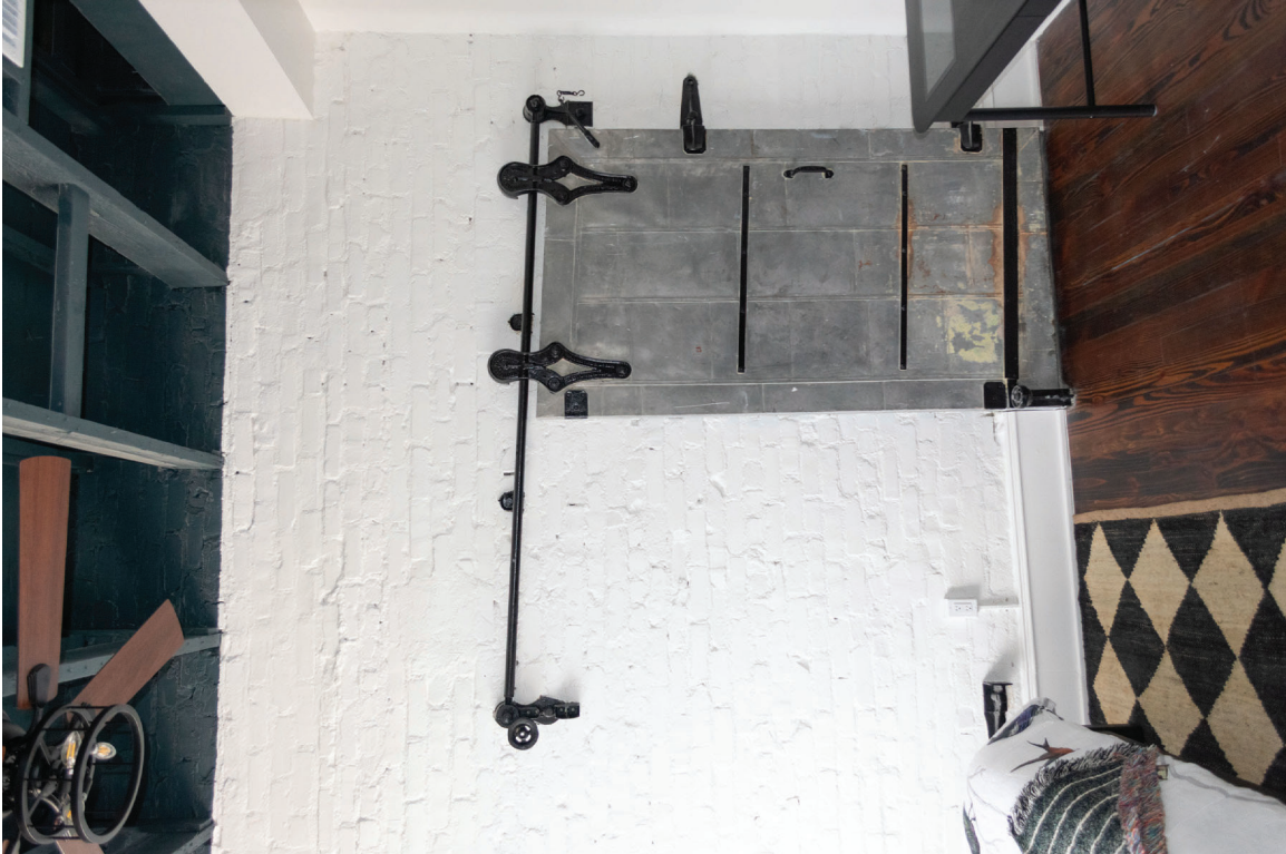
138 of 148: Interior, Room 225, historic fire door, photographer facing north.
