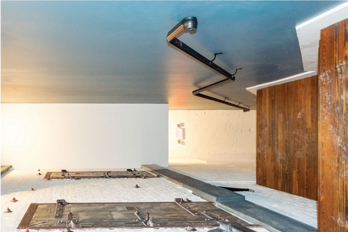
093 of 148: Interior, staircase, photographer facing west.
