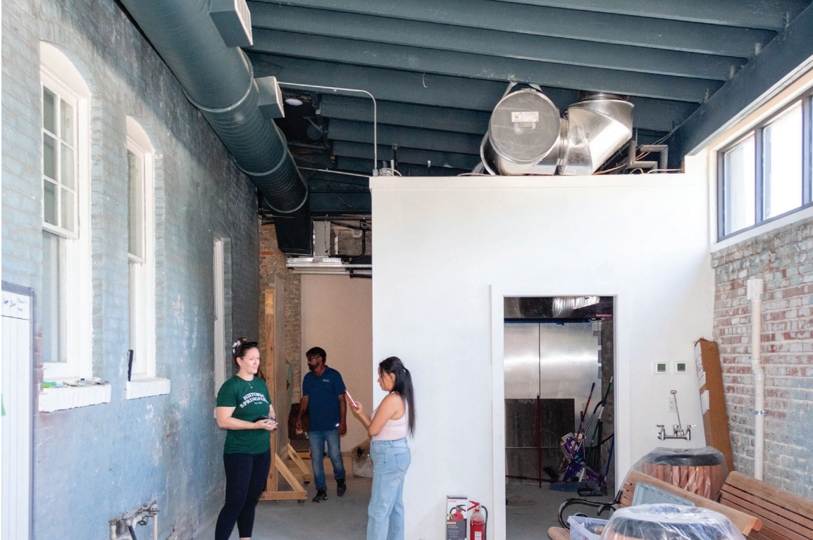
078 of 148: Interior, Room 114, photographer facing north.
