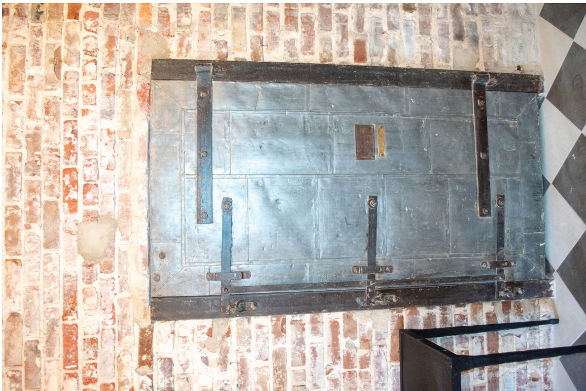
052 of 148: Interior, Room 100, photographer facing north.
