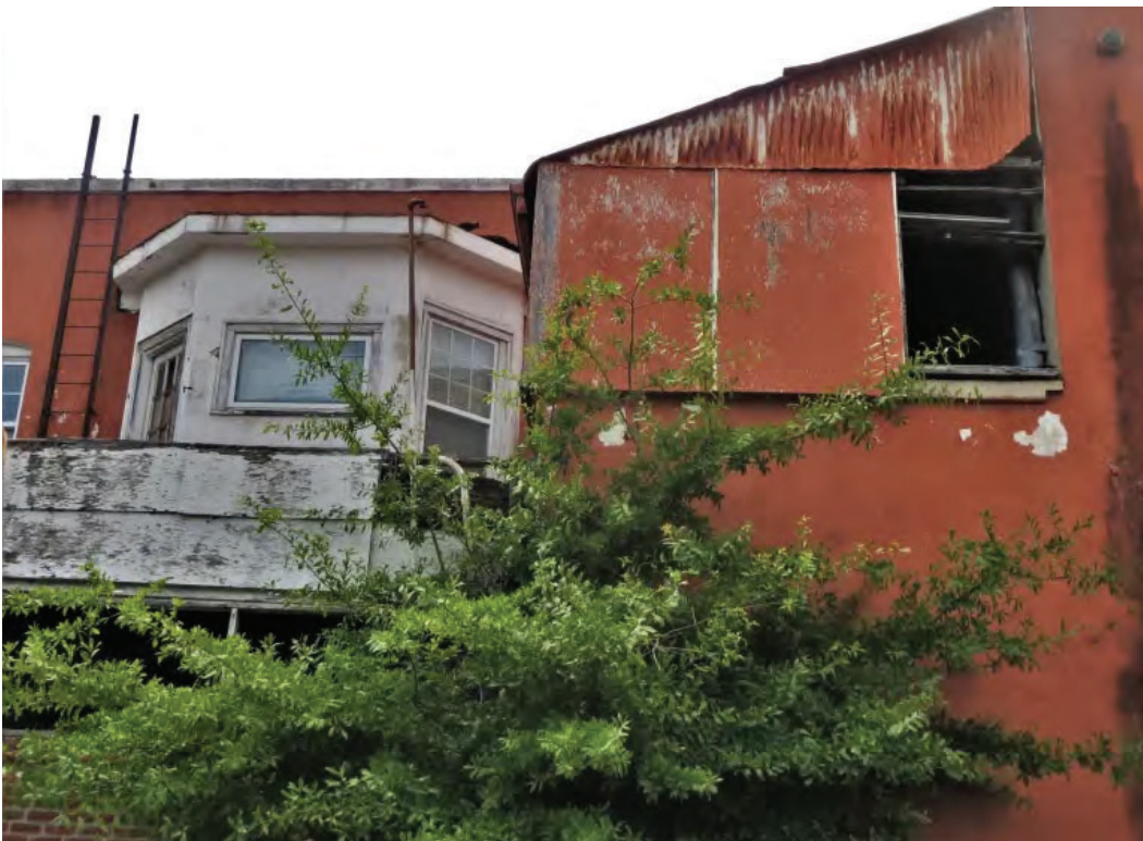
Figure 18: 2019 photograph of “bridge” between house and casket factory on second floo .
