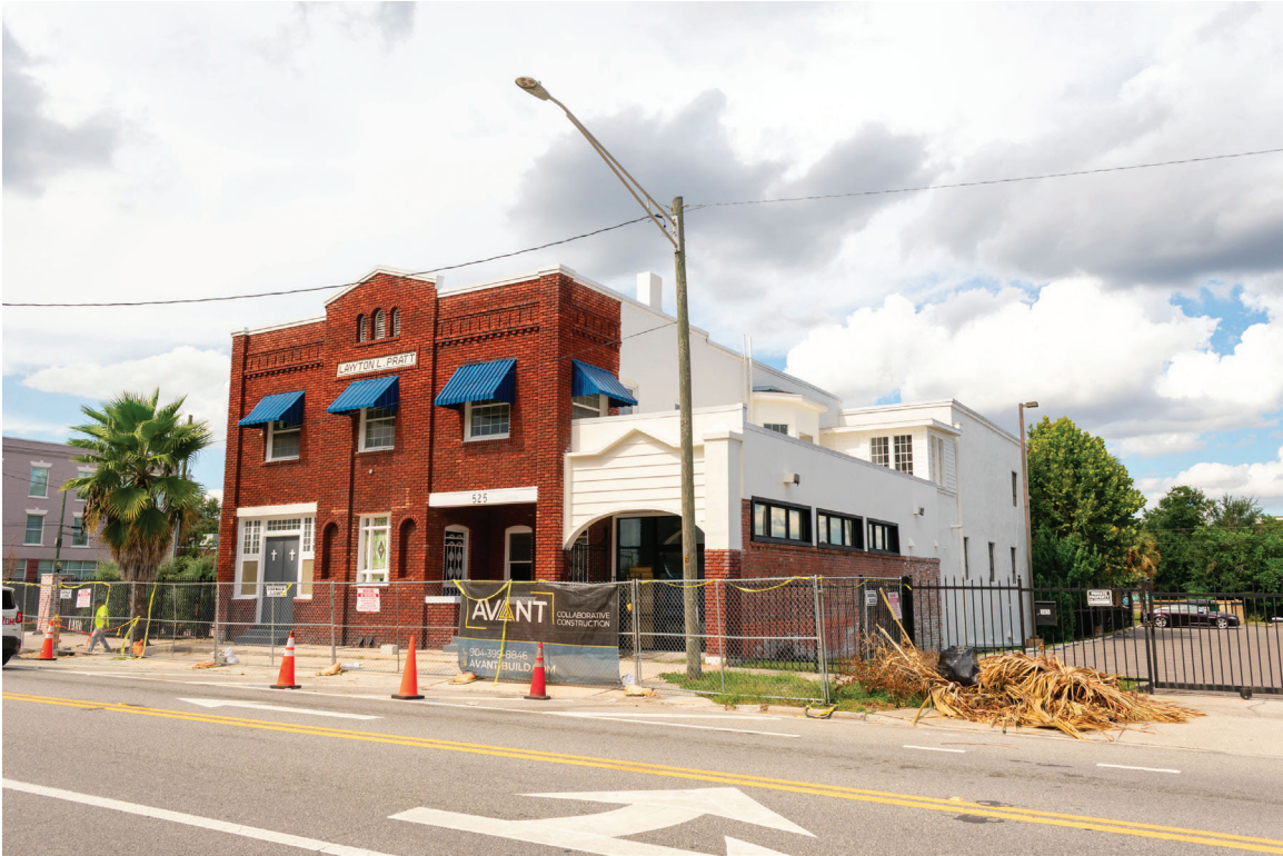
003 of 148: Exterior view, south (front) and east side elevations; photographer facing northwest.
