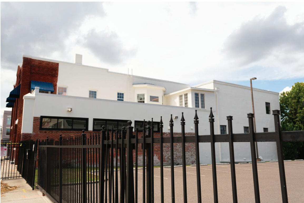
002 of 148: Exterior view, east side elevation; photographer facing northwest.
