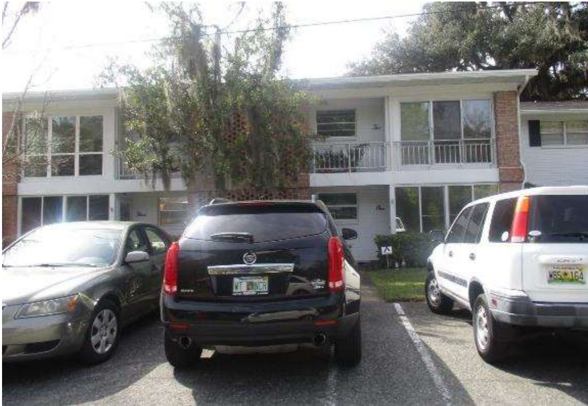
Adjacent multi-family structure
