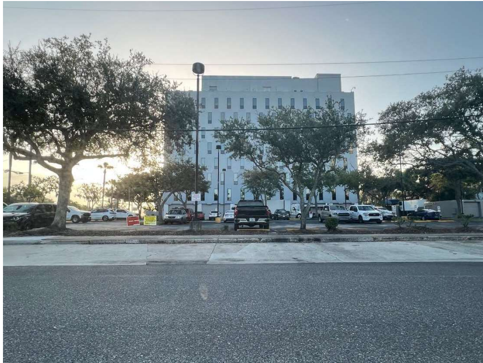
View of the existing office tower with the proposed hotel location in front
