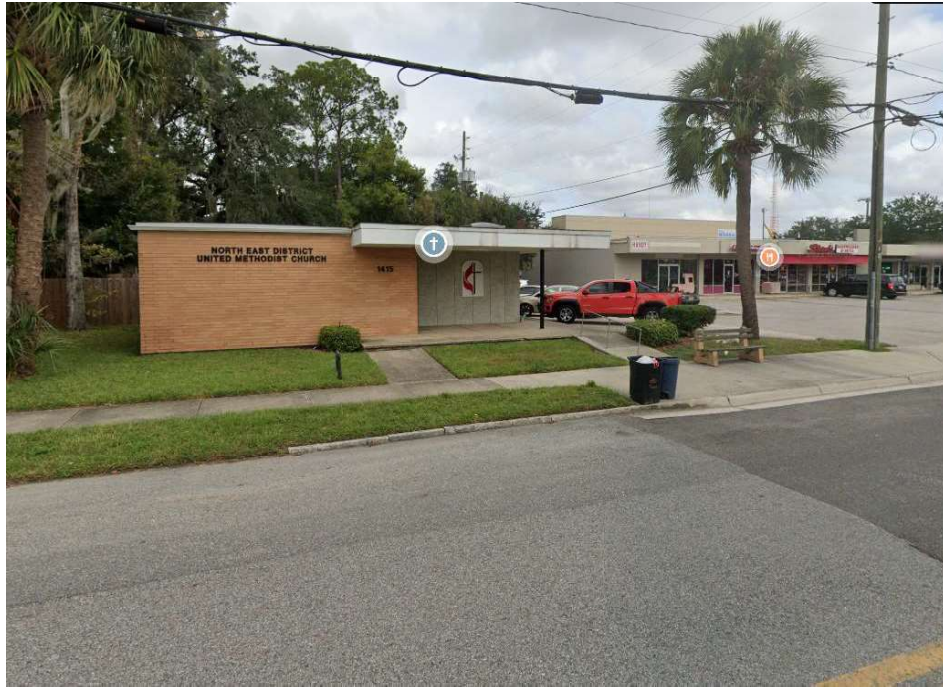
View of the Church looking towards the Subject Site
