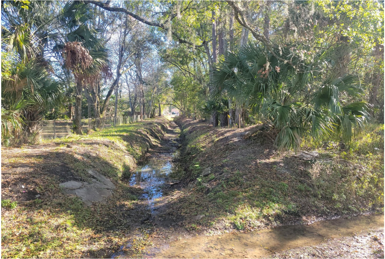
City owned drainageway to the north and east of the property.
