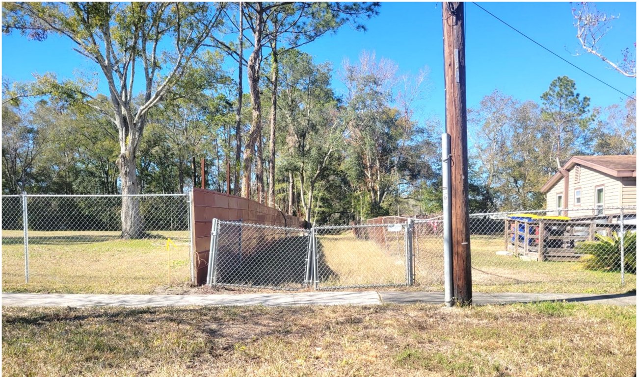
City owned drainageway to the east of the property facing north from Richardson Road.
