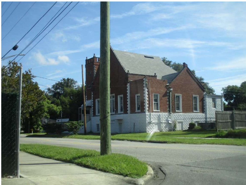
View of the neighboring church to the north
