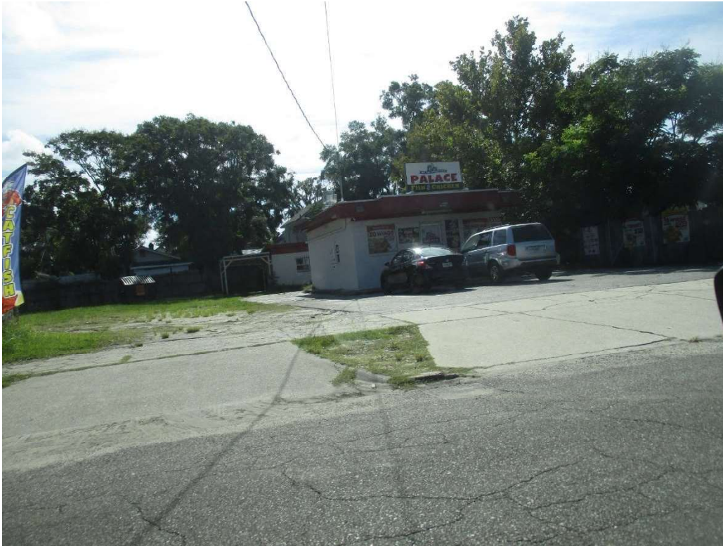
View of the neighboring restaurant to the south
