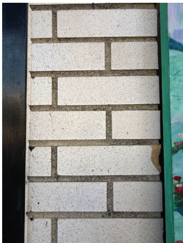
Photo 10: White Speckled Glazed Brick Closeup
