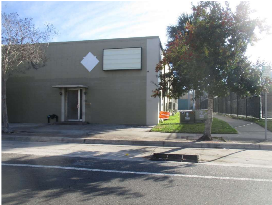
View of the Subject Site on the side closest to the Library
