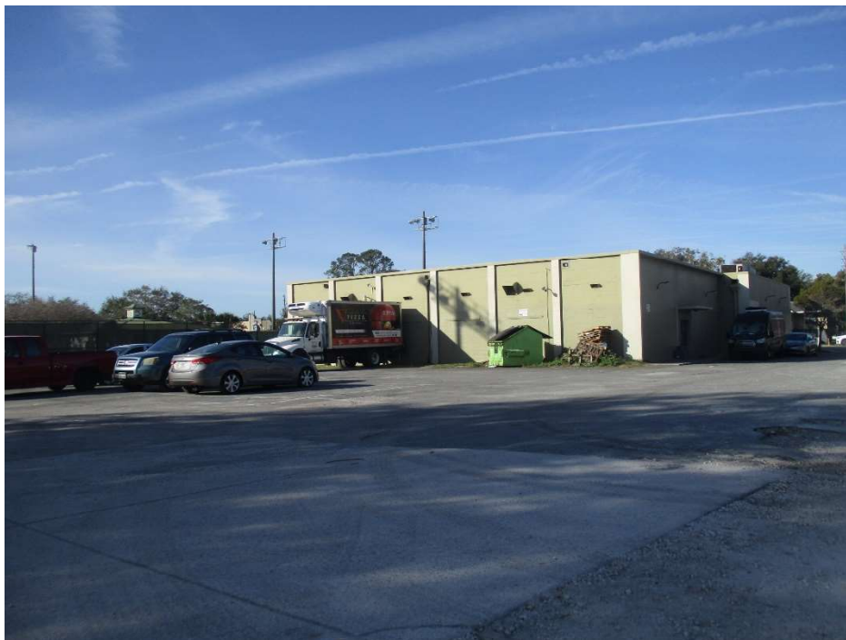
View of the City owned parking area behind the Subject Site
