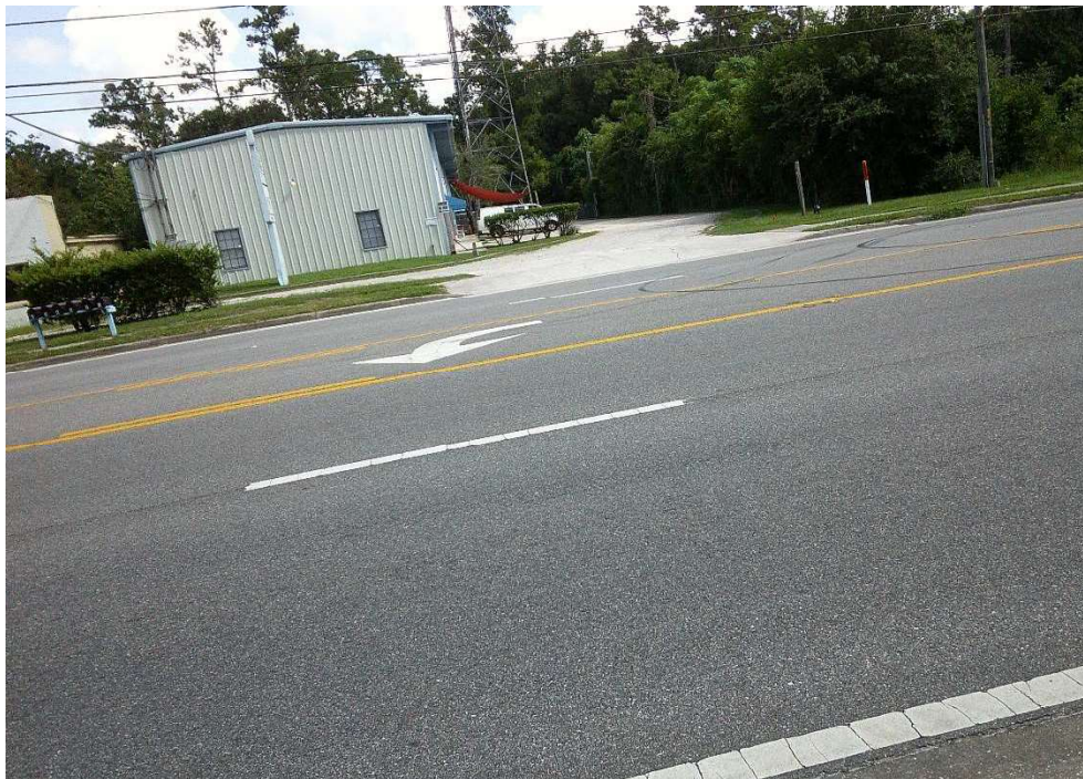
View of the warehouse use across Dunn Avenue
