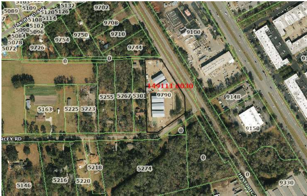
Source: Planning & Development Department, 5/30/2024 Aerial view of the subject property, facing north.
