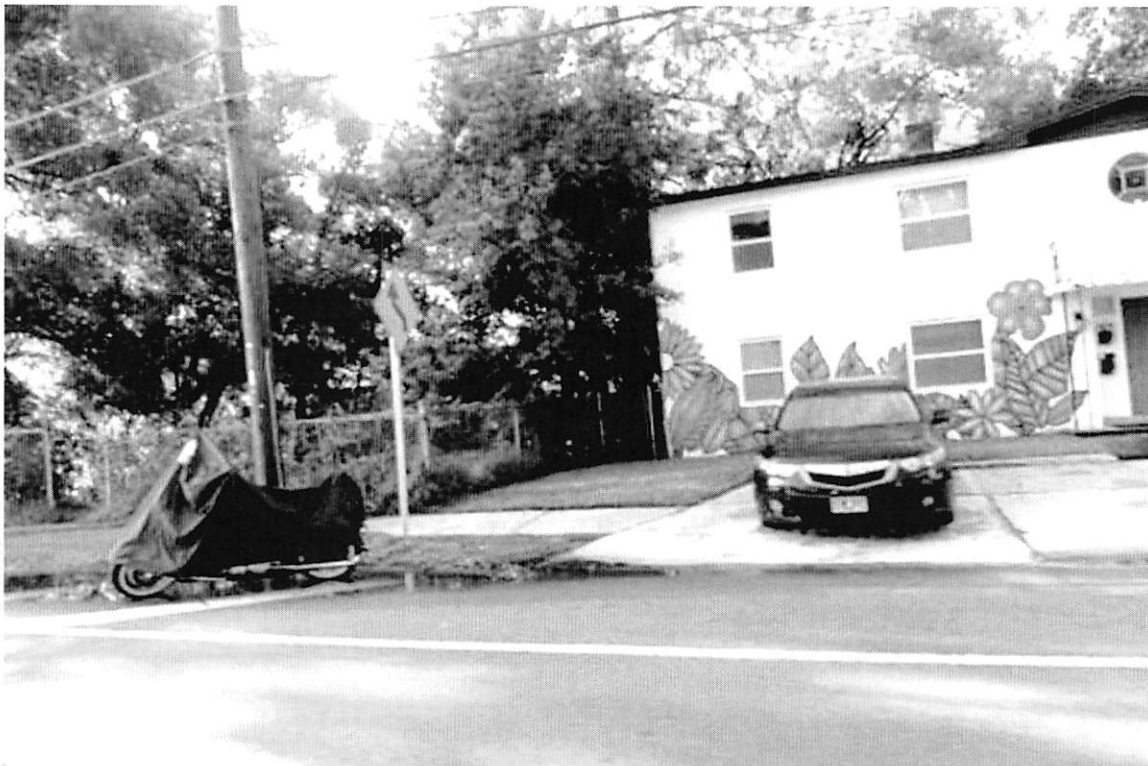
View of property on Post Street and adjacent multi-family
