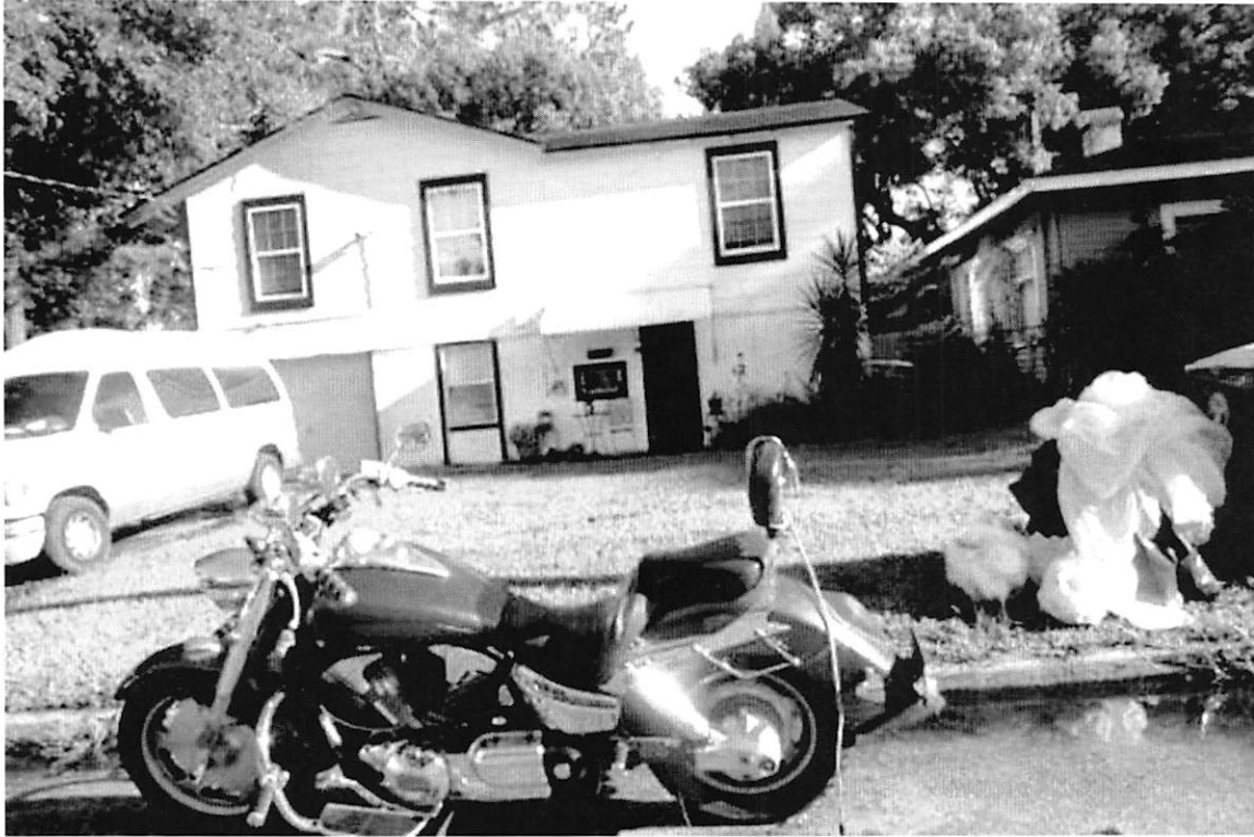
View of existing duplex on Cypress Street
