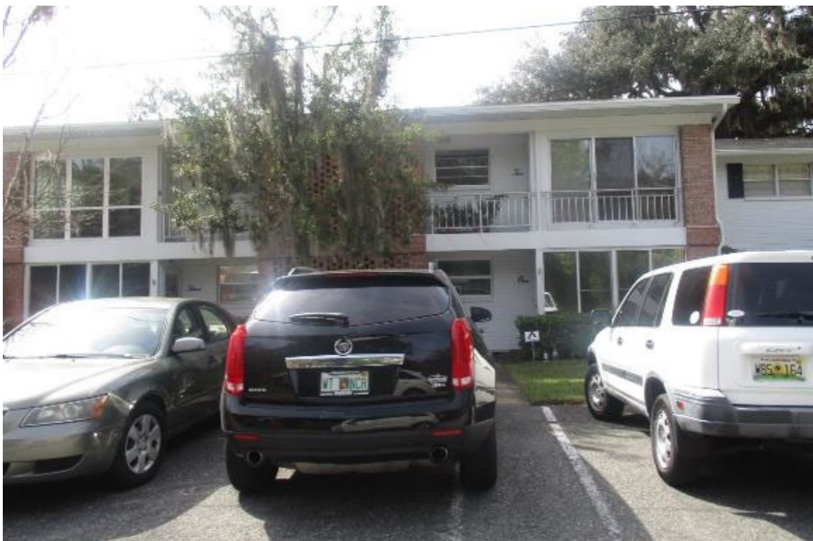
Adjacent multi-family structure
