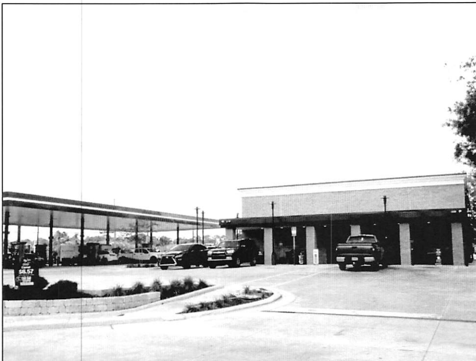
View of Property to the West
