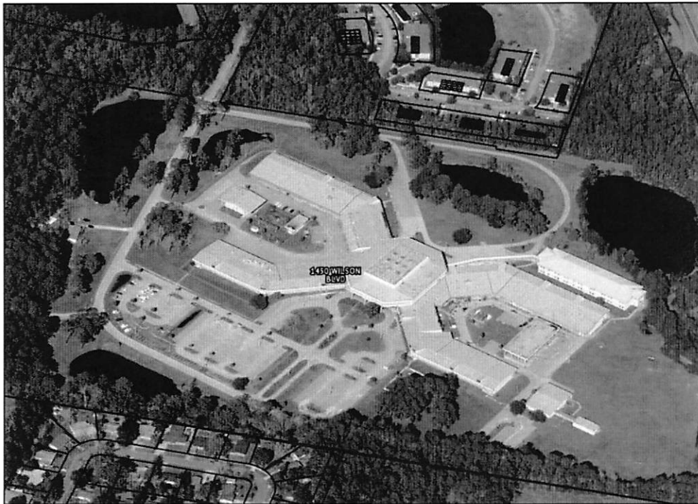
View of Property to the South
