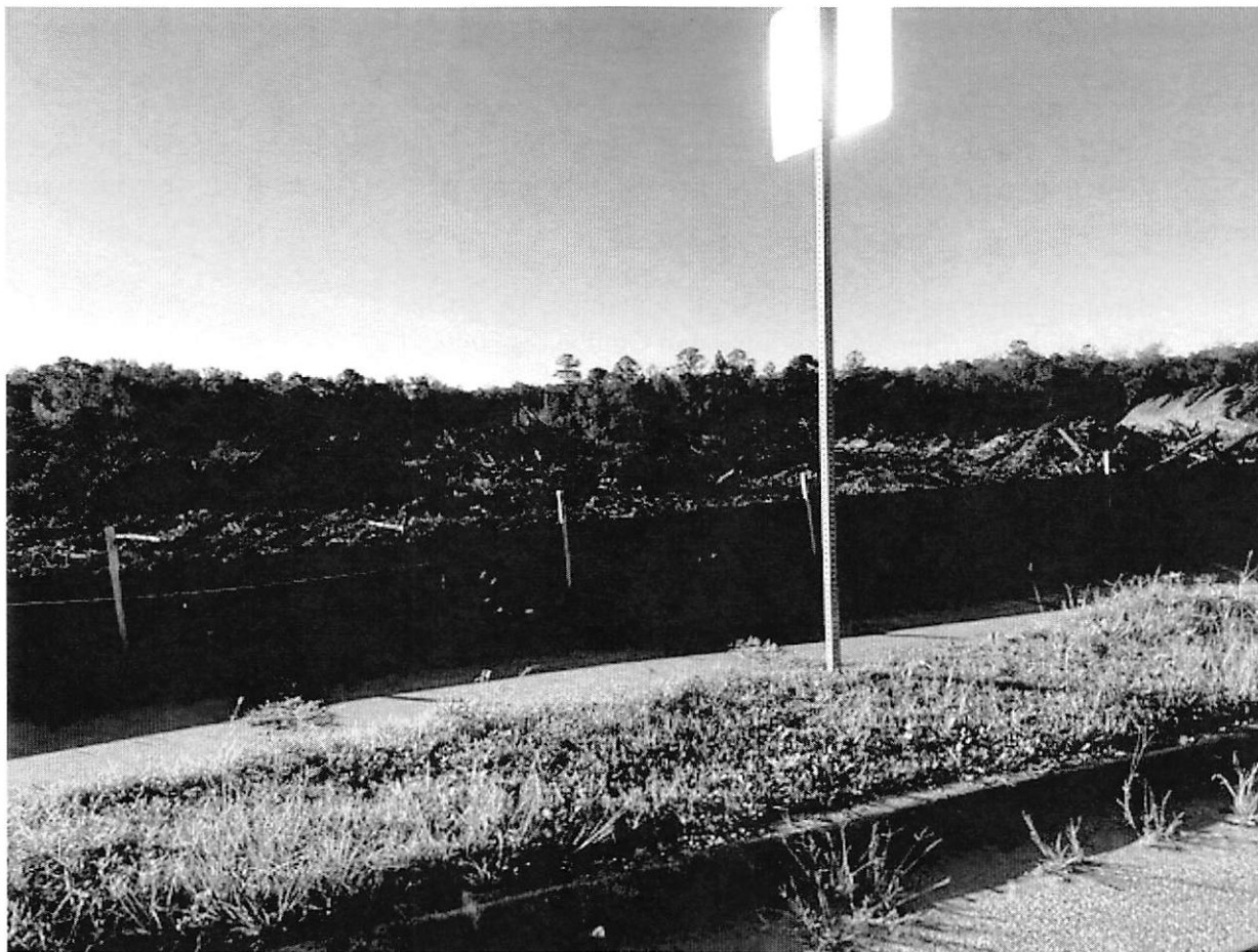
View of subject site being cleared.
