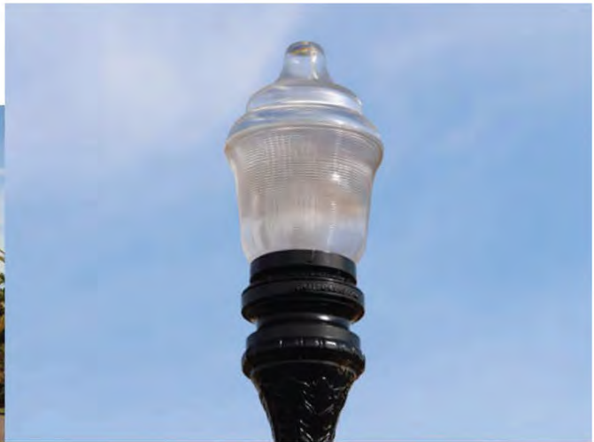
Figure 5.2 Examples of Plain Acorn Type Light Fixture (From JEA)
