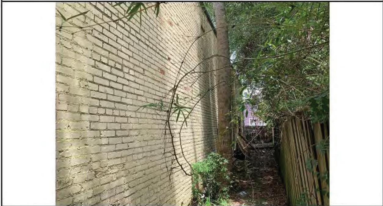
Photo 2: Partial southern elevation with wood fence to the right.
