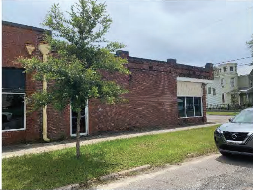
Photo 5: Partial northern elevation.
