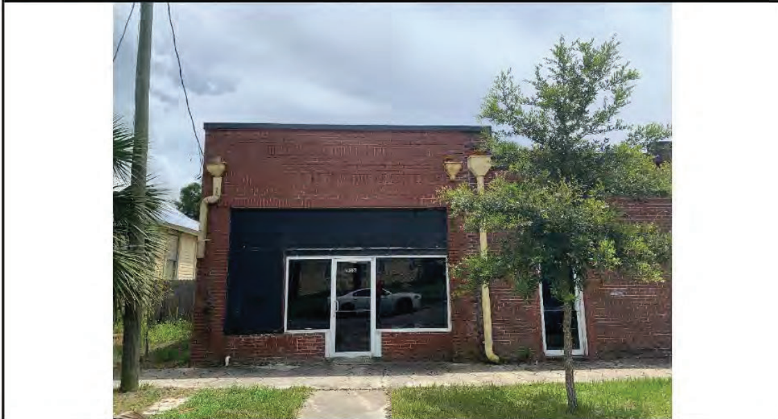
Photo 4: Partial northern elevation.
